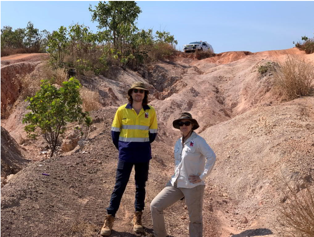
Figure 5-11: Erosion from 4WD tracks to Gunn Point Beach
