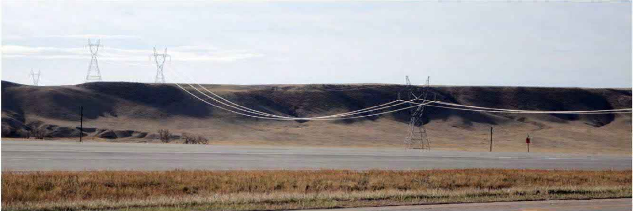
Figure 8–10: View wires that have not been selected or treated for non-reflectivity. This is to be avoided (Source: Bureau of Land Management, 2013)
