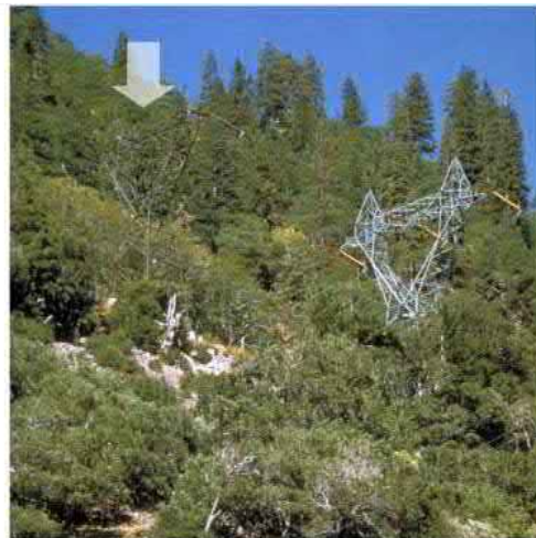
The color-treated lattice tower to the upper left of the untreated tower blends in very well with the surrounding landscape, and could easily be missed by a casual viewer. (Credit: John McCarty, BLM.)
