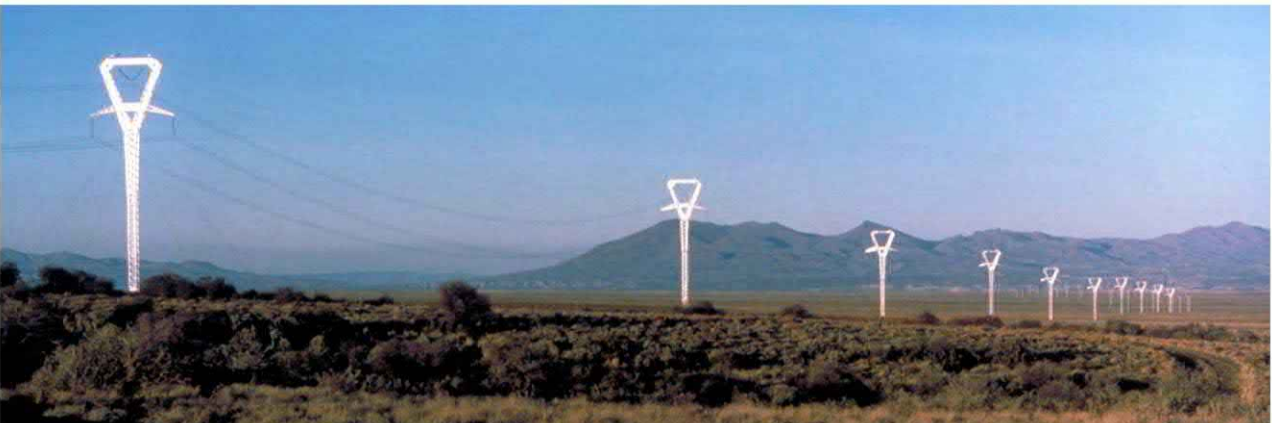
Figure 8-9: View showing conspicuous reflective transmission line viewed against a mountain backdrop (Source: Bureau of Land Management, 2013)
