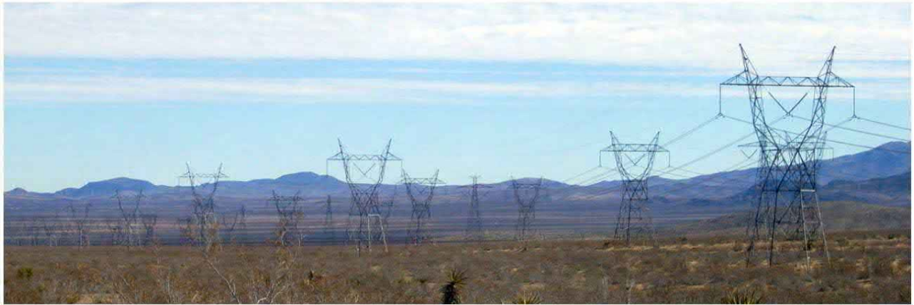
Figure 8–3: Collocation of transmission lines reduces overall visual impact (Source: Bureau of Land Management, 2013)
