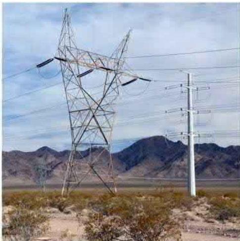
Weathered lattice tower and white monopole. An additional lattice tower is visible in the background to the left of the large lattice tower. (Credit: Robert Sullivan, Argonne National Laboratory.)
