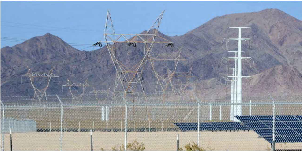
Figure 8-8: View showing the difference visual prominence of lattice towers versus monopoles (Source: Bureau of Land Management, 2013)
