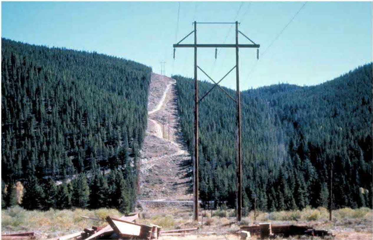
Figure 8–5: View showing how the bisection of a ridgeline can create a conspicuous linear element in the landscape (Source: Bureau of Land Management, 2013)
