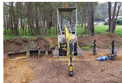
1.7 T CAT excavator on tracks (different accessories) for secondary channels
