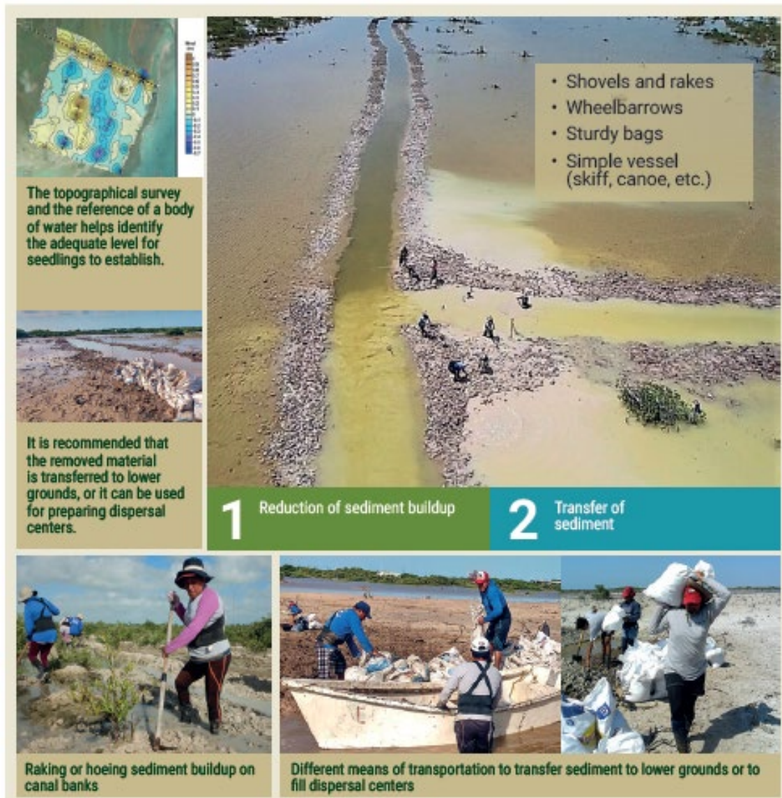
Figure 3-3 Steps and recommendations for sediment removal for the topography rehabilitation.
