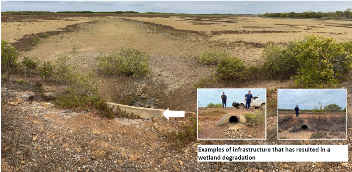
Figure 3-9 BC-S2C team looking at culverts requiring rehabilitation
