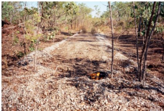
Plate 7. North Australian railway, facing south
