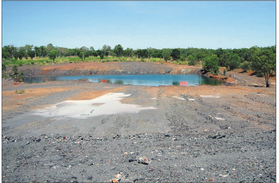
Plate 7.7 Partially backfilled trial pit (March 2005)
