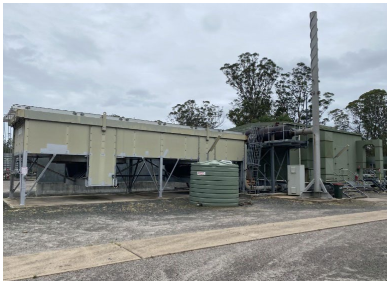
Figure 30: Indicative Compressor Package, including compressor unit and fin fan cooler
