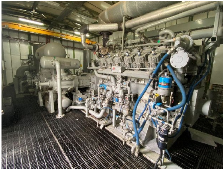
Figure 32: Indicative gas compressor drive engine
