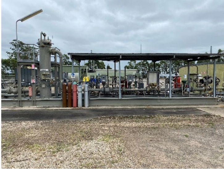
Figure 35: Indicative sales gas metering skid
