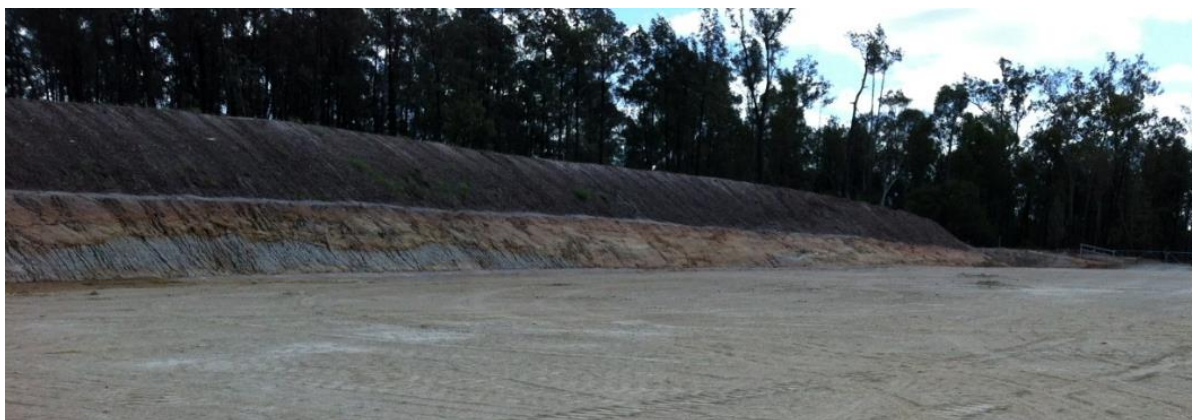
Figure 5.3—3 Topsoil Windrow Used to Divert Clean Water Away from the Well Pad
