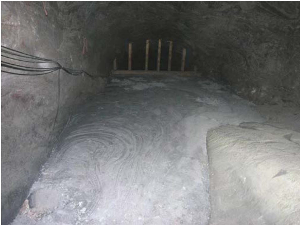
Figure 7-4 Hydraulic backfill using viscous slurry technique
