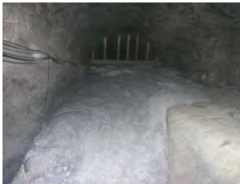
Plate 3-9 Typical underground hydraulic backfill
