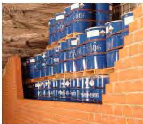
Plate 3-7 Example of simple single-skin wall seal in
