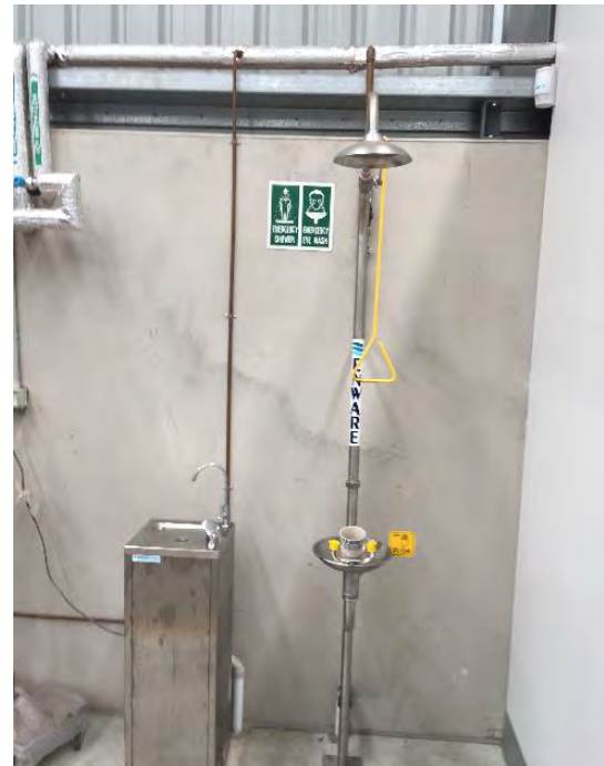
Plate 3-11 Example of emergency shower and eye wash station
