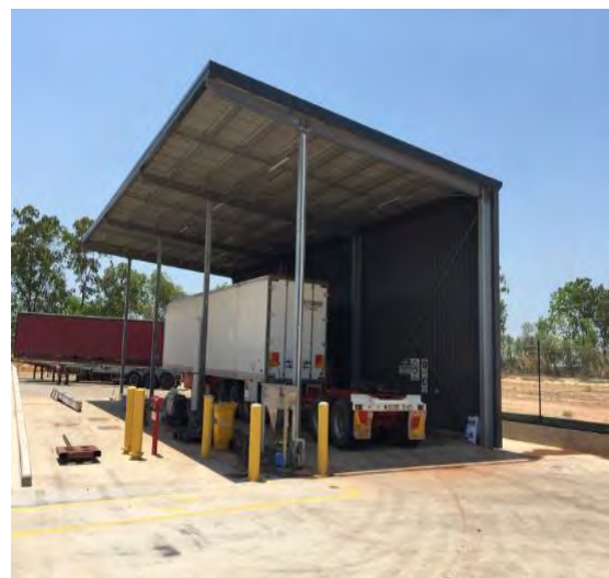
Plate 3-14 Example of vehicle wash down facility
