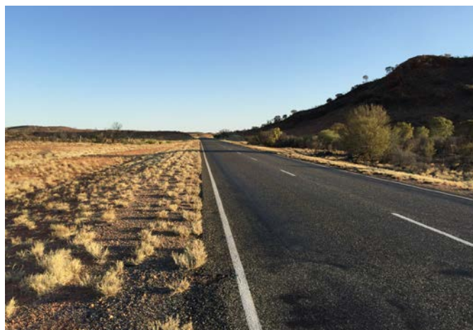
Plate 18-3 The Stuart Highway (in the vicinity of the proposed T-intersection at Henbury Access Road)
