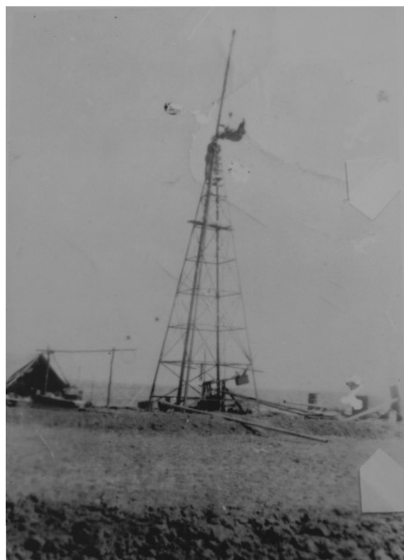
Plate 2. 'D' pattern windmill nearing completion, Ucharonidge Station. (source: Coral Beebe)
