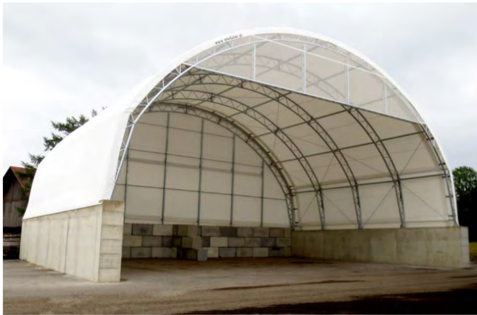
Figure 2-17. Example of the Petcoke storage area
