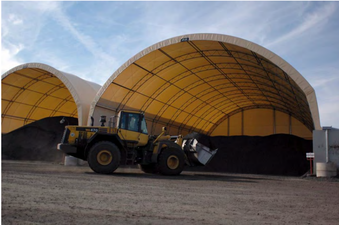
Figure 2-13. Example of Concentrate Storage Shed
