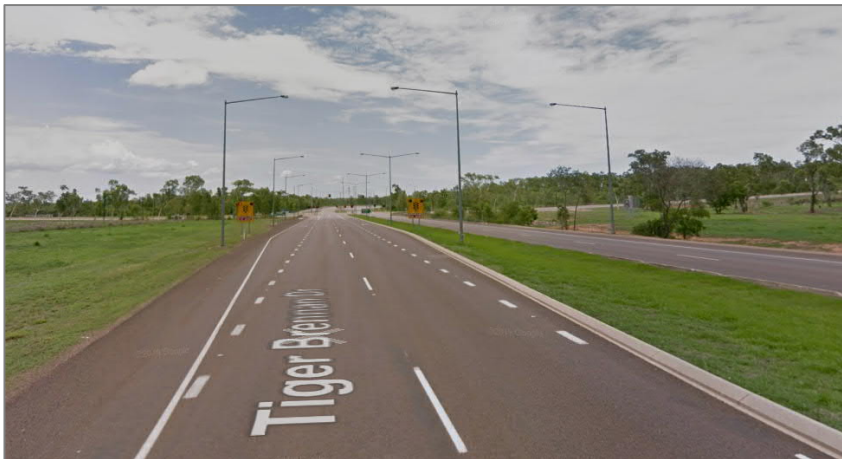
Figure 6 Tiger Brennan Drive intersection with Berrimah Road, view to the west
