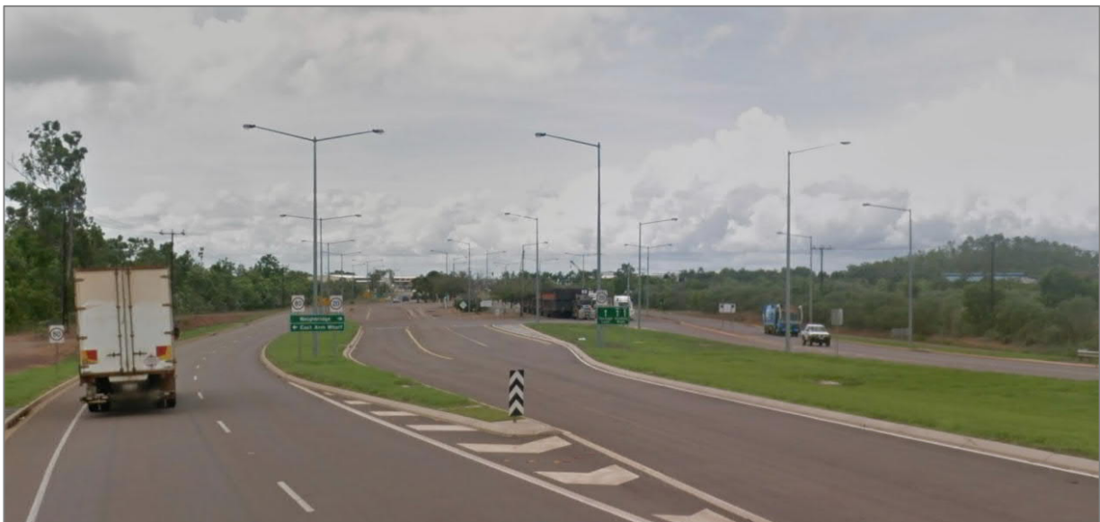
Figure 5 Berrimah Road South of Wishart Road intersection, view to the south
