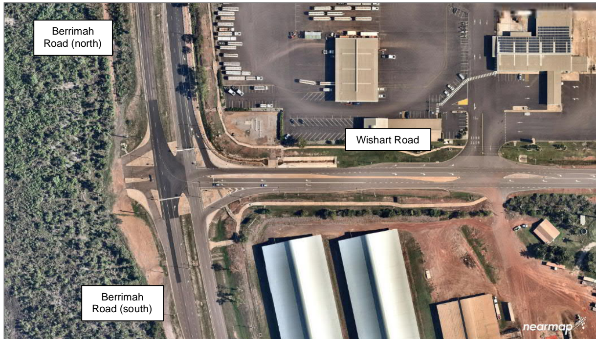
Figure 12 Aerial image of the Berrimah Road and Wishart Road intersection
