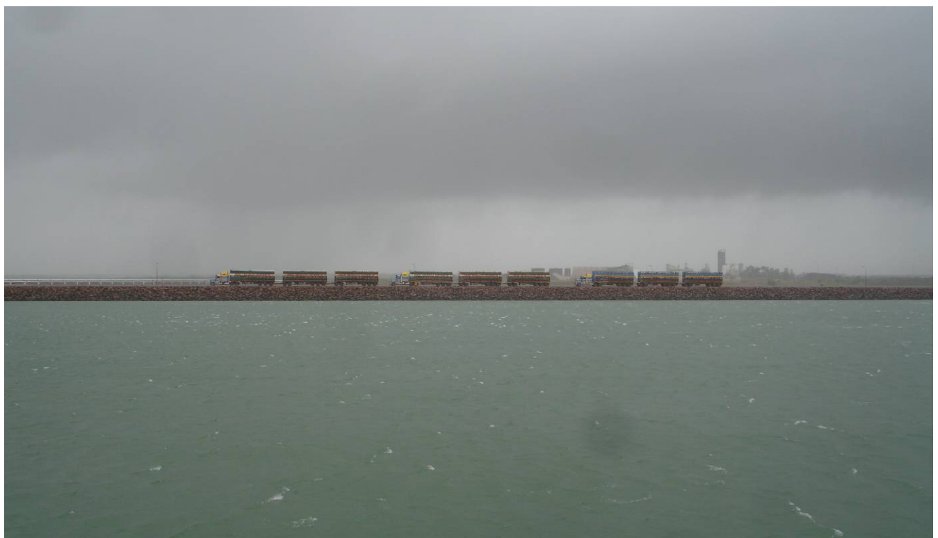
Figure 4 Top: EAW access road looking westward; Bottom: Looking westward towards access road from new hardstand area
