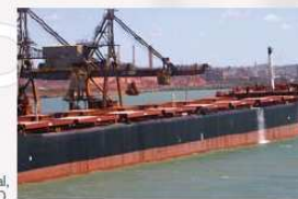
Port loading terminal, Gladstone QLD.
