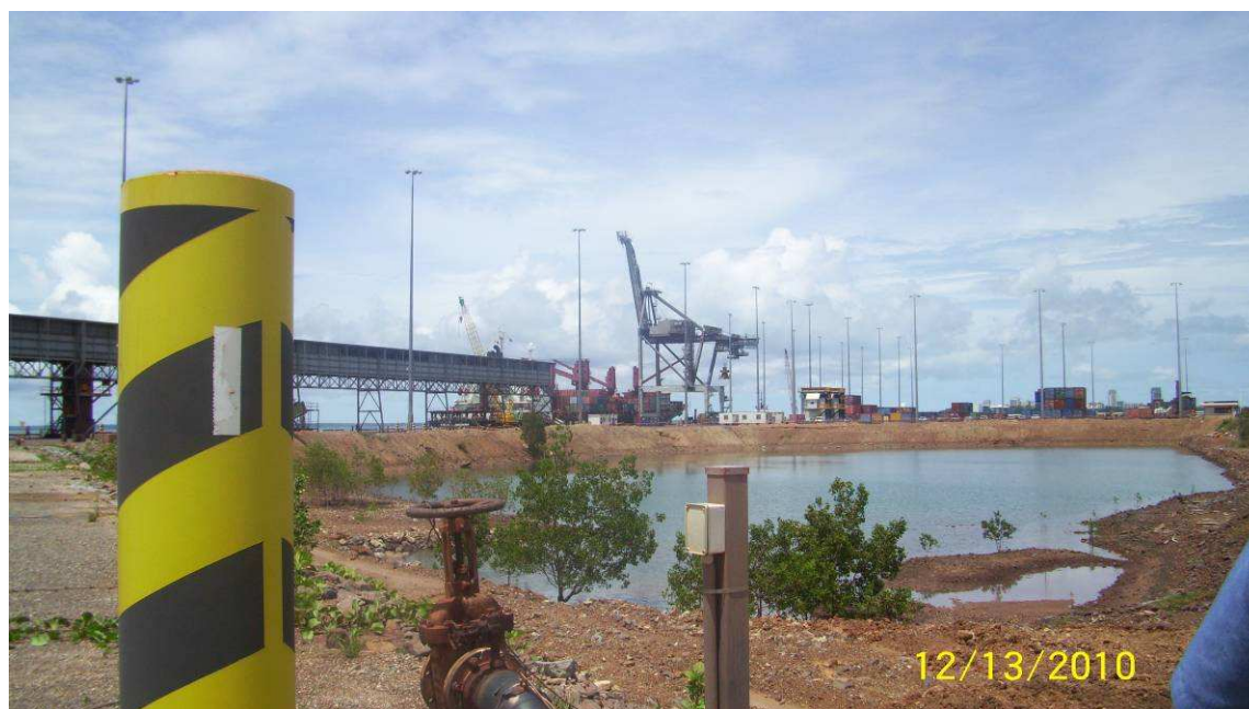
Figure 3 Pond F at EAW looking southward
