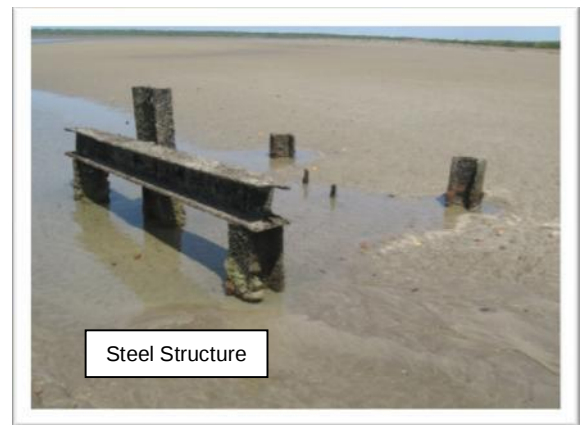
Figure 15 Photograph of the unidentified steel structure
