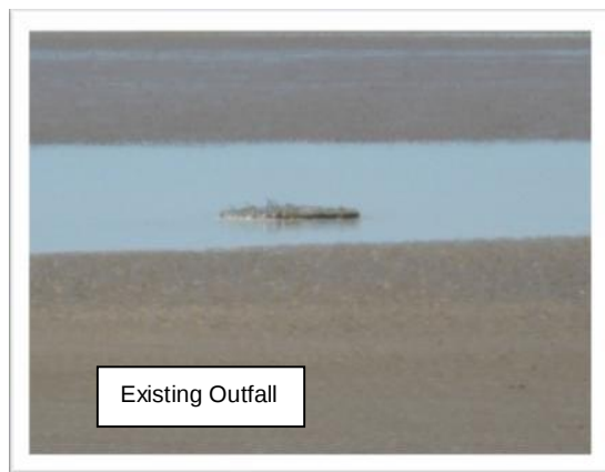
Figure 14 Photograph of the existing East Point outfall
