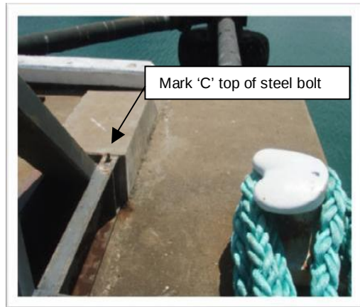
Figure 4 Benchmark on Fort Hill Wharf. (Elevation = 5.892mAHD)
