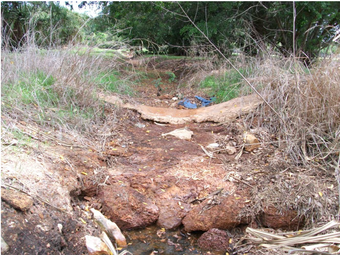
Photo 6: Very dense laterite exposed in a drain cutting adjacent to BH27.
