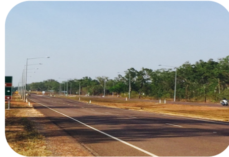
Intersection at Stuart Highway and Cox Peninsula Road, from Stuart Highway
