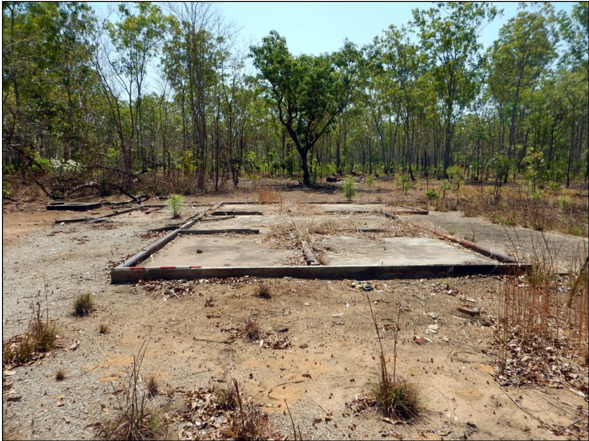
Figure 6. Site 1 – Slab 1. Foundations and slab. Scale in 20cms.
