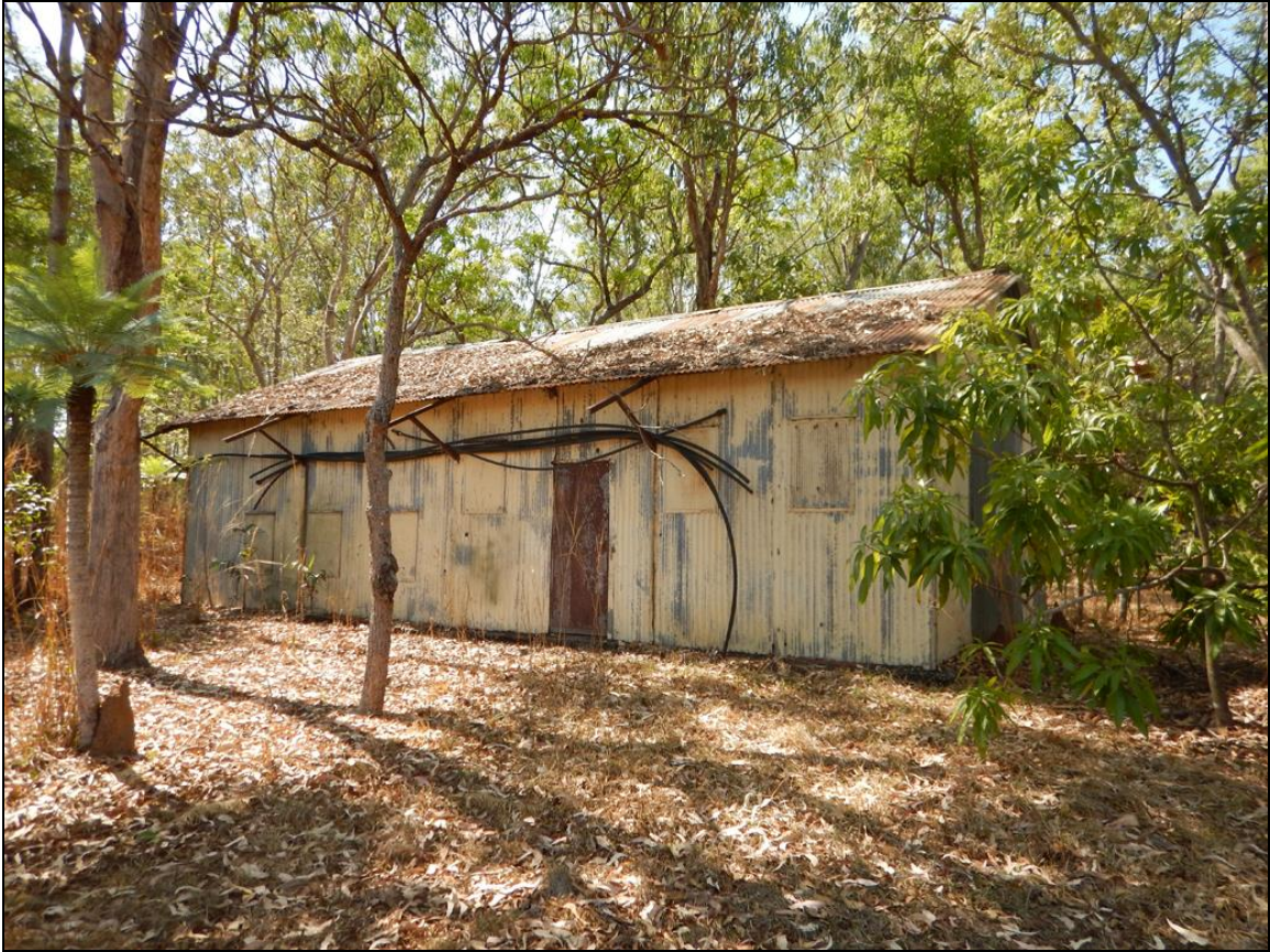
Figure 3. Sidney Williams shed near Site 3.
