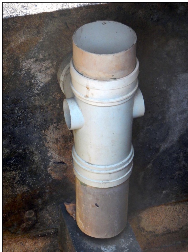
Figure 8. Site 1 – Slab 1. Septic tank PVC plumbing.
