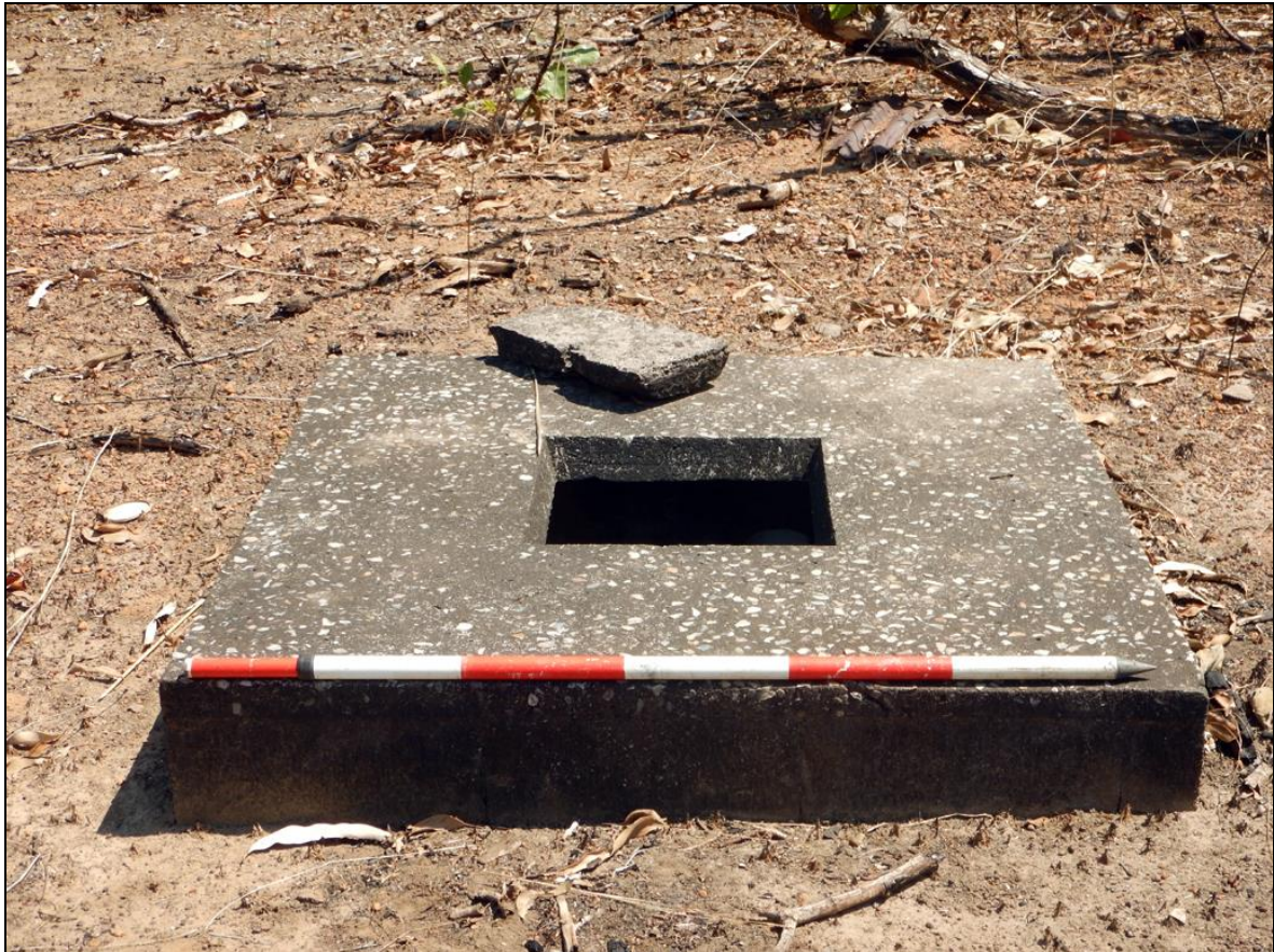
Figure 7. Site 1 – Slab 1. Septic tank. Scale in 20cms.
