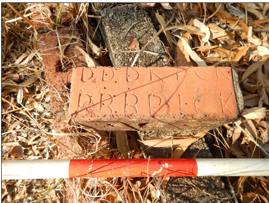
Figure 25. Site 3 brick with 'B.B. Brick' imprint. Note: double brick wall. Scale in 20cms.
