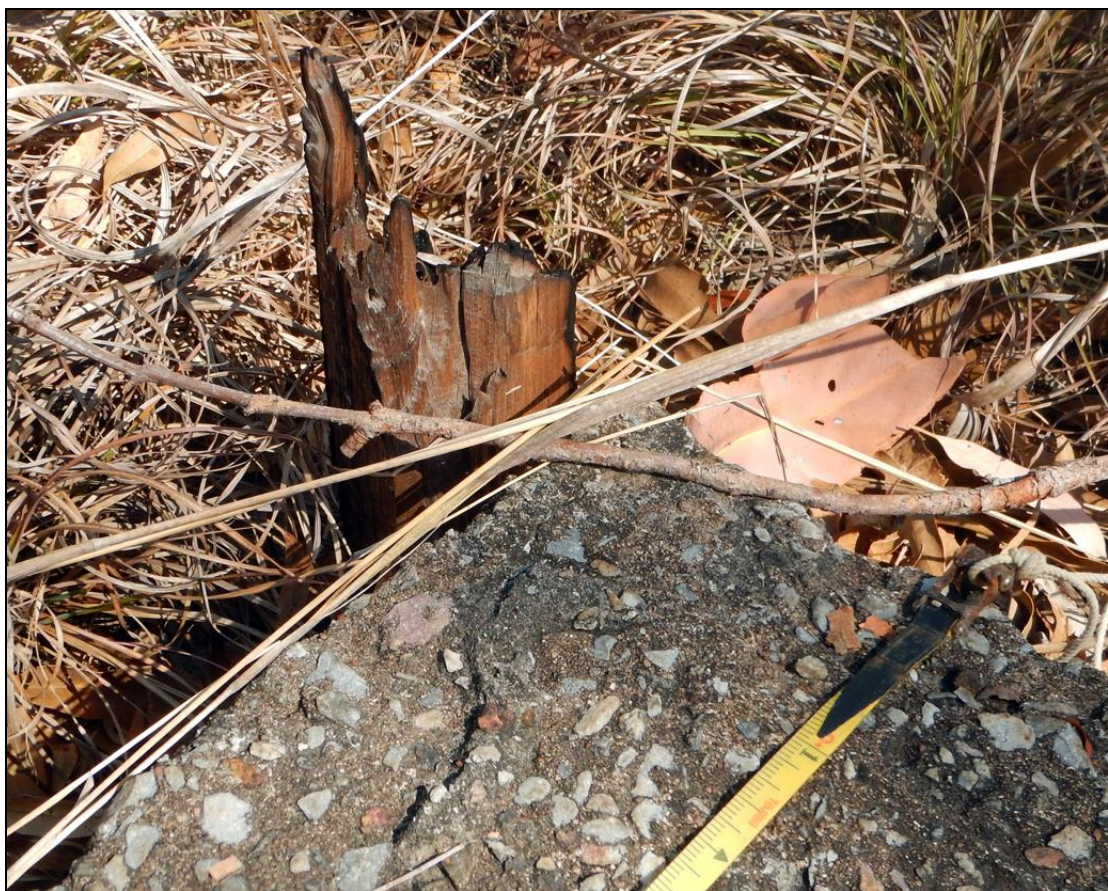
Figure 15. Site 2 – Slab 3. Wood formwork. Scale in 1cms.
