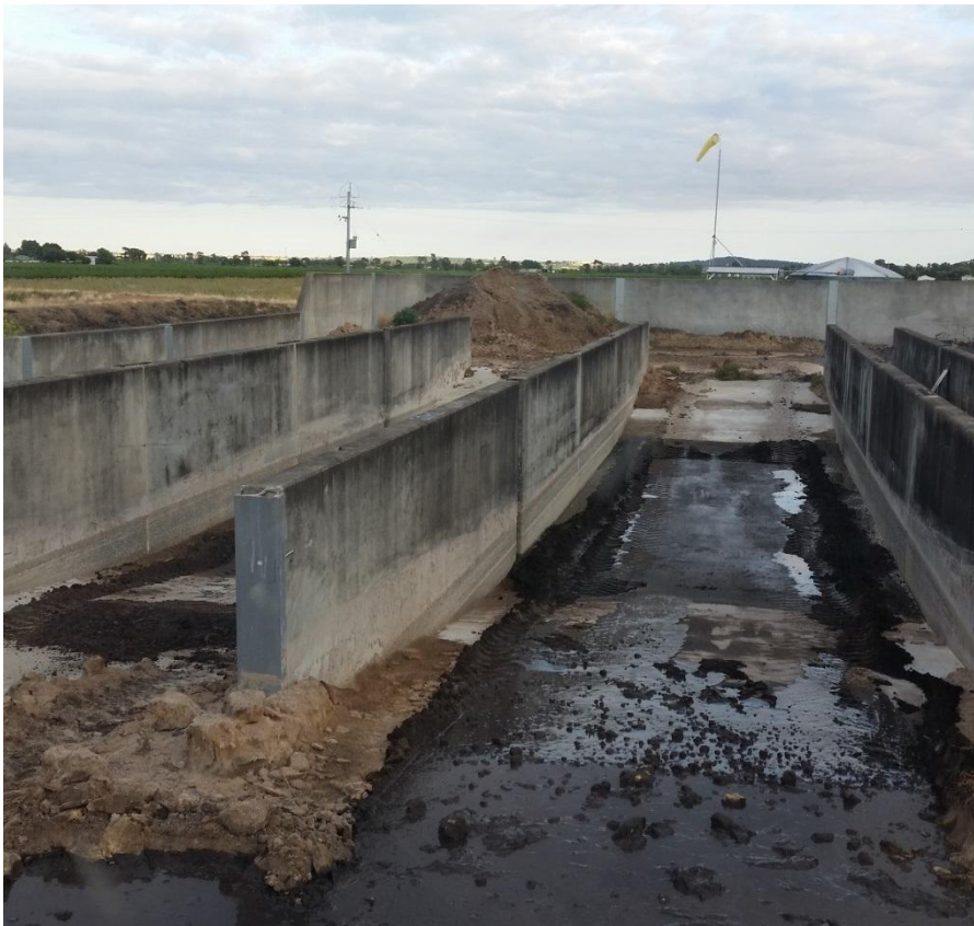
Figure 12 Concrete sedimentation terrace
