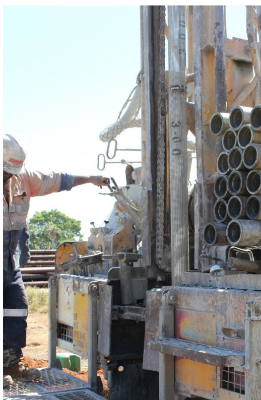
Figure 11 Stainless Steel wire wound screen placed to 113m
