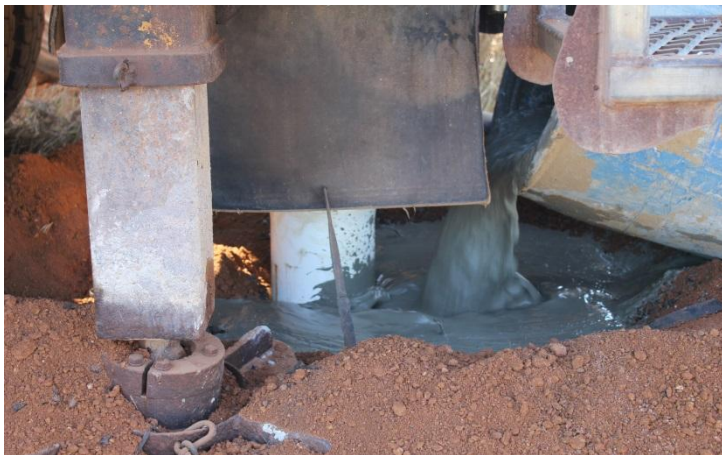
Figure 8 Grout sealing of surface casing
