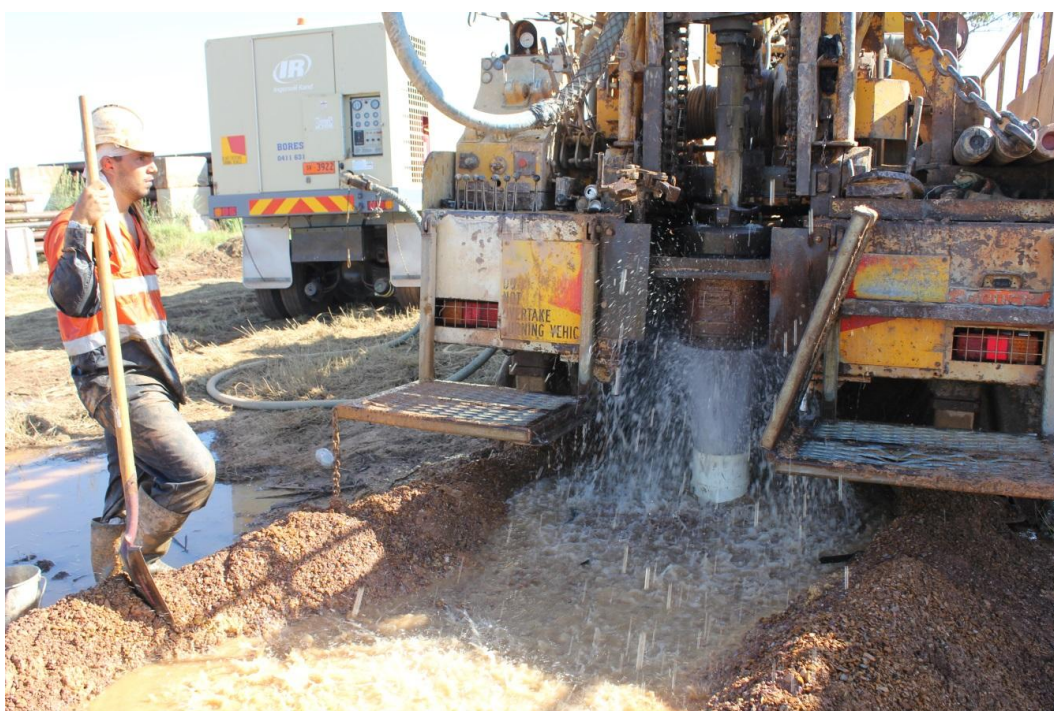
Figure 4 RAB Drilling in operation with Water Strike
