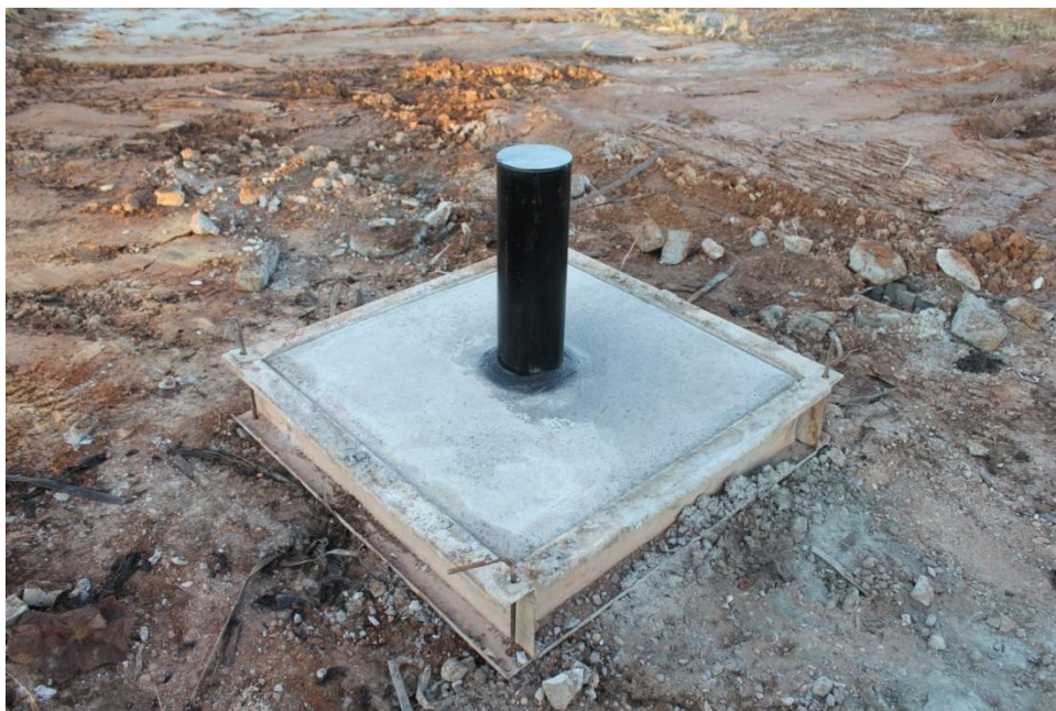
Figure 14 Concrete collar and slab with 152mm ID Casing extending above ground
