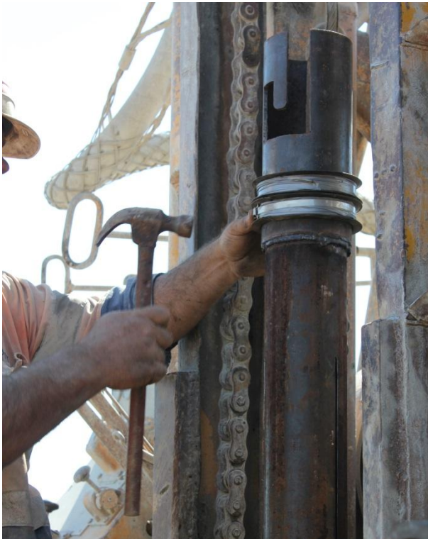
Figure 12 Installation of Casing
