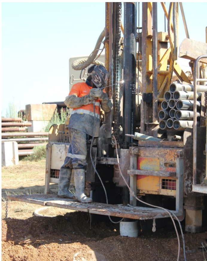
Figure 10 Welding 152mm ID Steel Casing String
