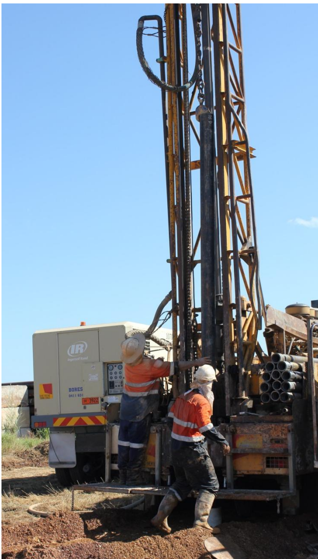
Figure 9 Installation of 4.8m slotted casing (screen) placed to 71.2m
