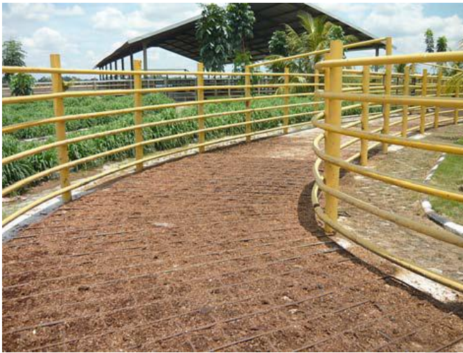
Figure 18 Concrete Paved High Traffic Areas
