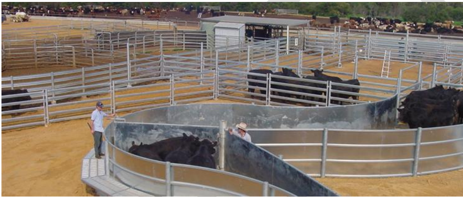
Figure 14 Cattle Handling Facilities
