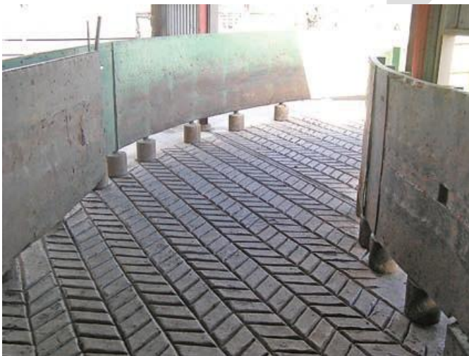
Figure 19 Concrete Paved Cattle Handling Areas
