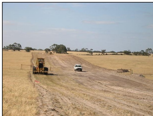
Grading of pipeline corridors. W. Mathieson/Ecos
