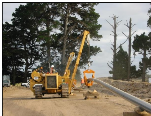
Pipe being lowered into the trench Ecos
