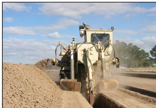
Trenching machine in action Ecos
