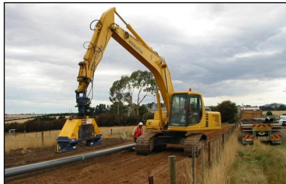
Pipe stringing. Ecos
