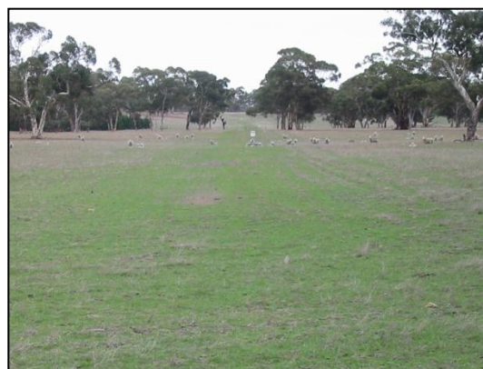
An operational pipeline corridor. Ecos
