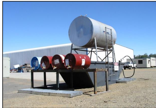
Temporary storage of fuel and oils at a yard/campsite. Ecos
