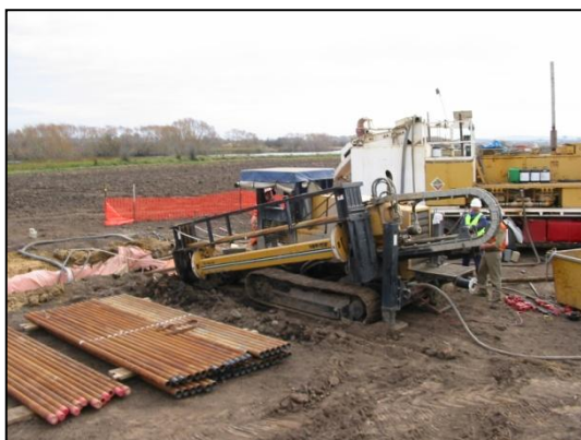
Small horizontal directional drilling rig. Ecos
