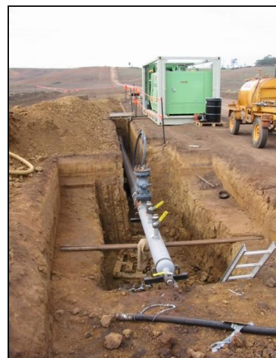
Hydrostatic testing a section of pipeline. Ecos
