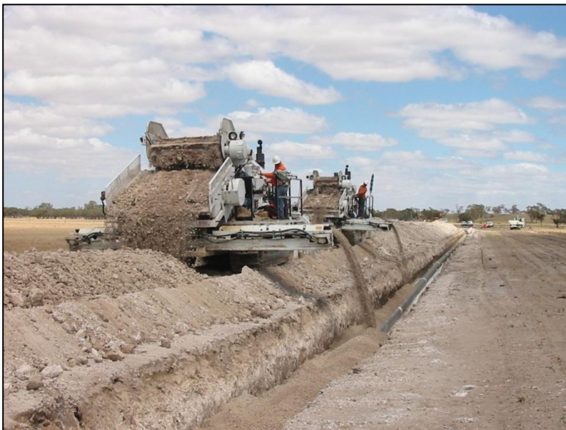
Padding machine returning spoil to the trench. Ecos
