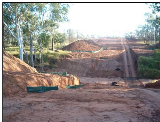
Erosion controls (berms and sediment fences) at a watercourse crossing. W. Mathieson
