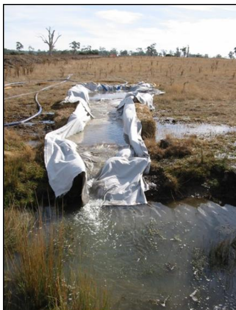
Erosion controls at a trench de-watering site. Ecos
