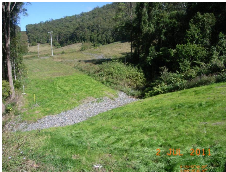
Rehabilitation on a large diameter pipeline RoW – CNC Project Management
