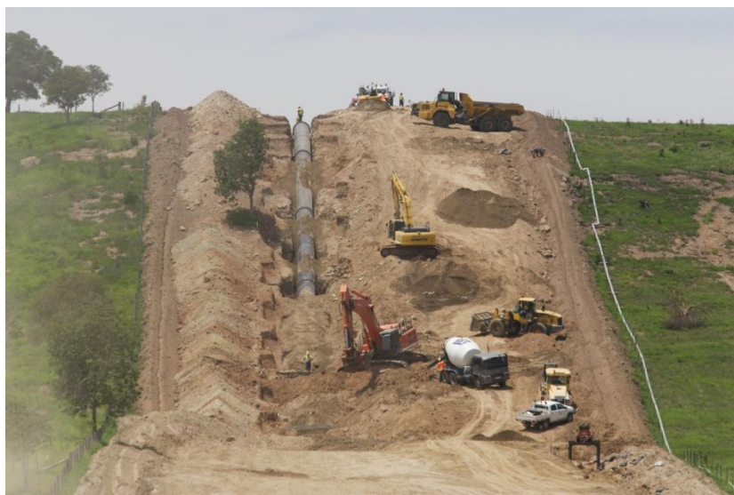
Typical pipeline construction corridor for a large transmission pipeline (>800 mm diameter). MacDow
