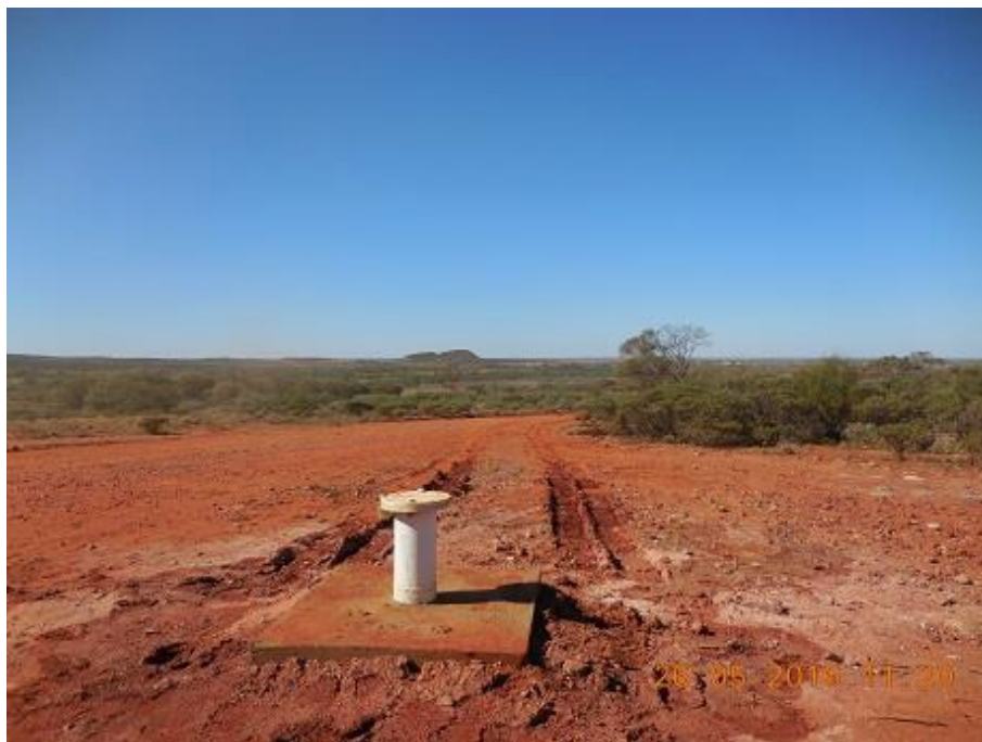
Figure 1 – Example of flanged monitoring bore completion
