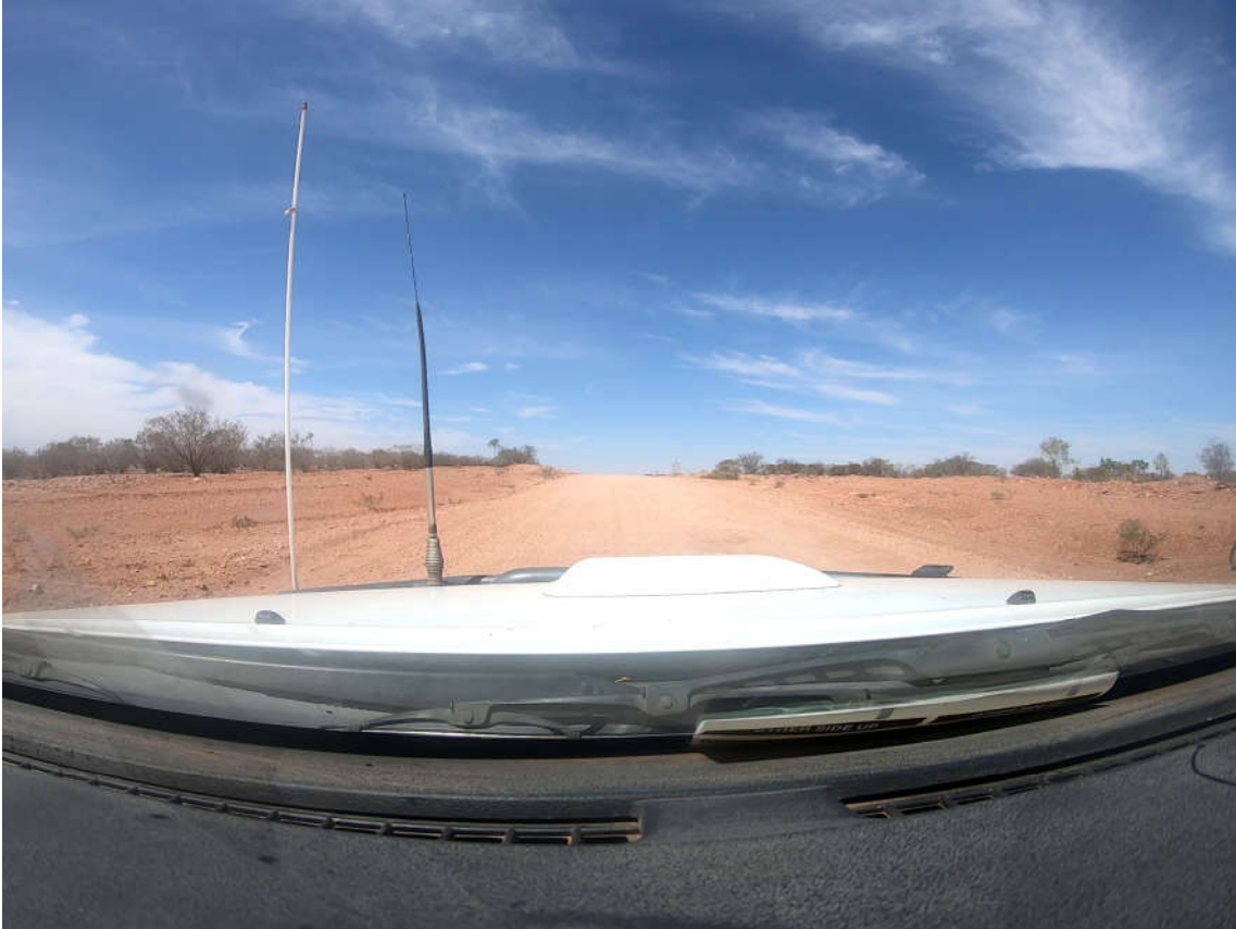
Photo 10 – Insufficient sight distance to crest at Ch. 229.09km
