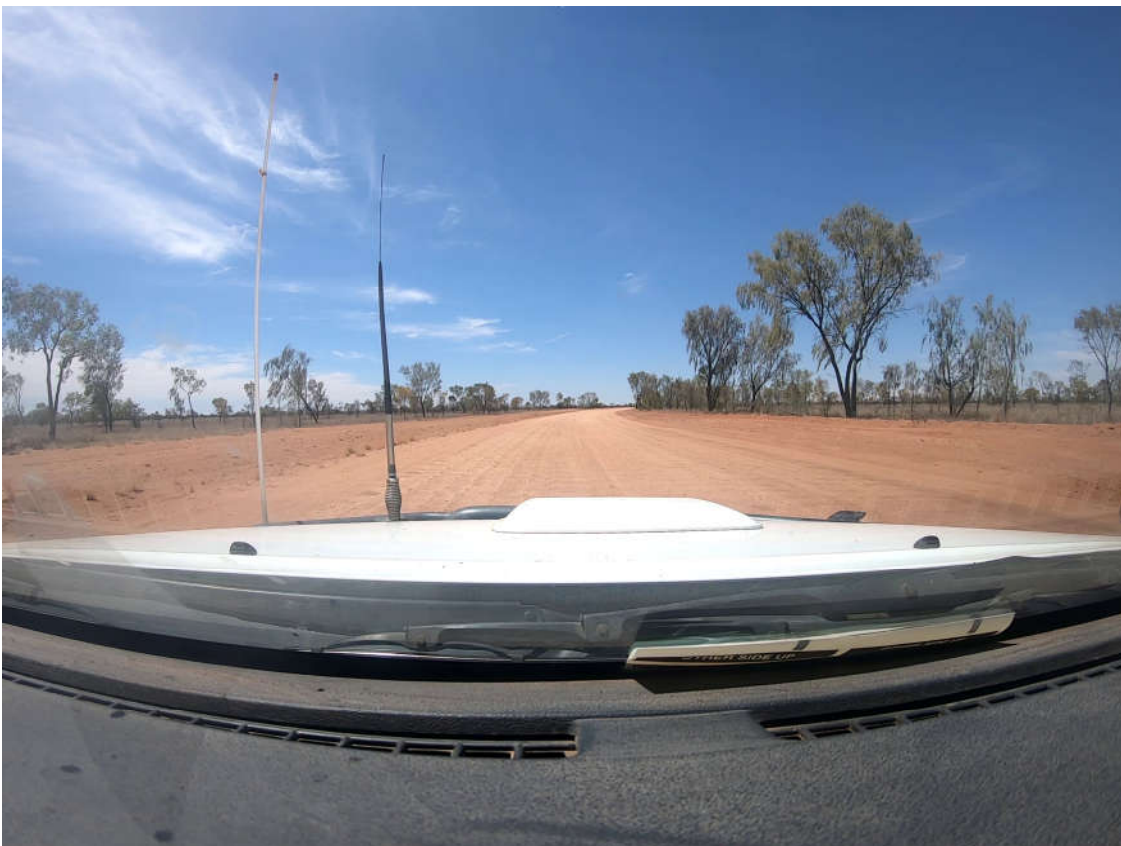
Photo 7 – Trees block sight distance through horizontal curve
