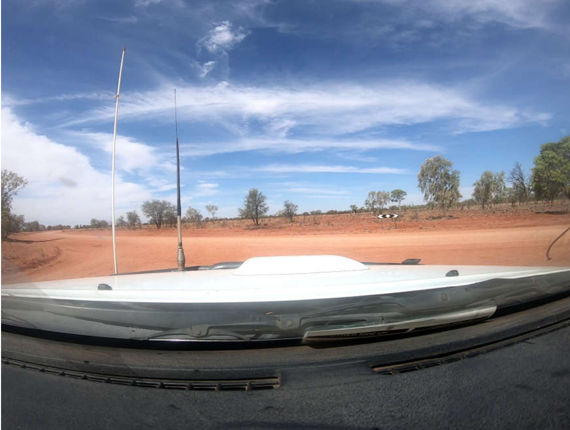
Photo 14 – Insufficient sight distance to Jervois intersection
