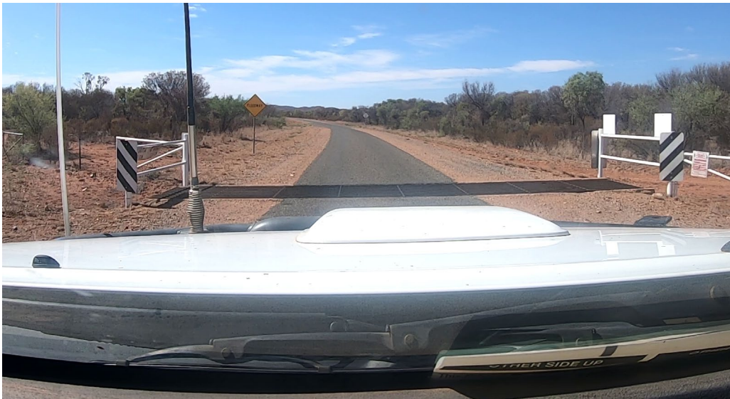
Photo 3 - Single Lane Seal and Gravel Shoulders
