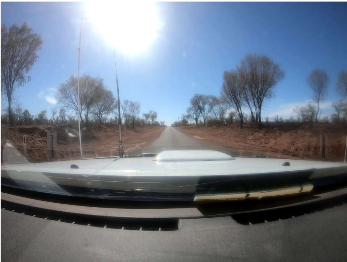
Photo 4 – Poor sight distance
