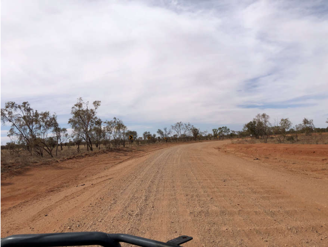
Photo 16 – Sub-standard horizontal curve immediately before Lucy Creek Access
