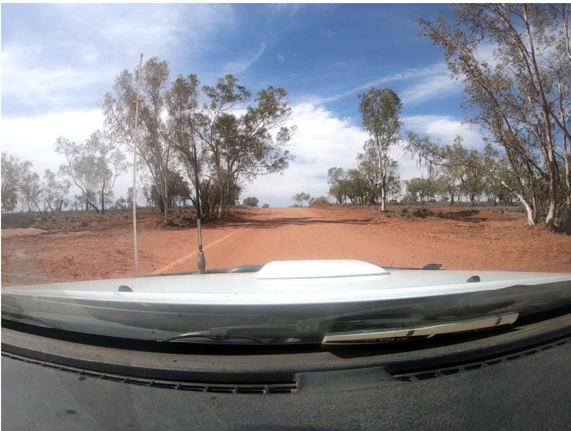
Photo 13 – Poor sight distance to crest
