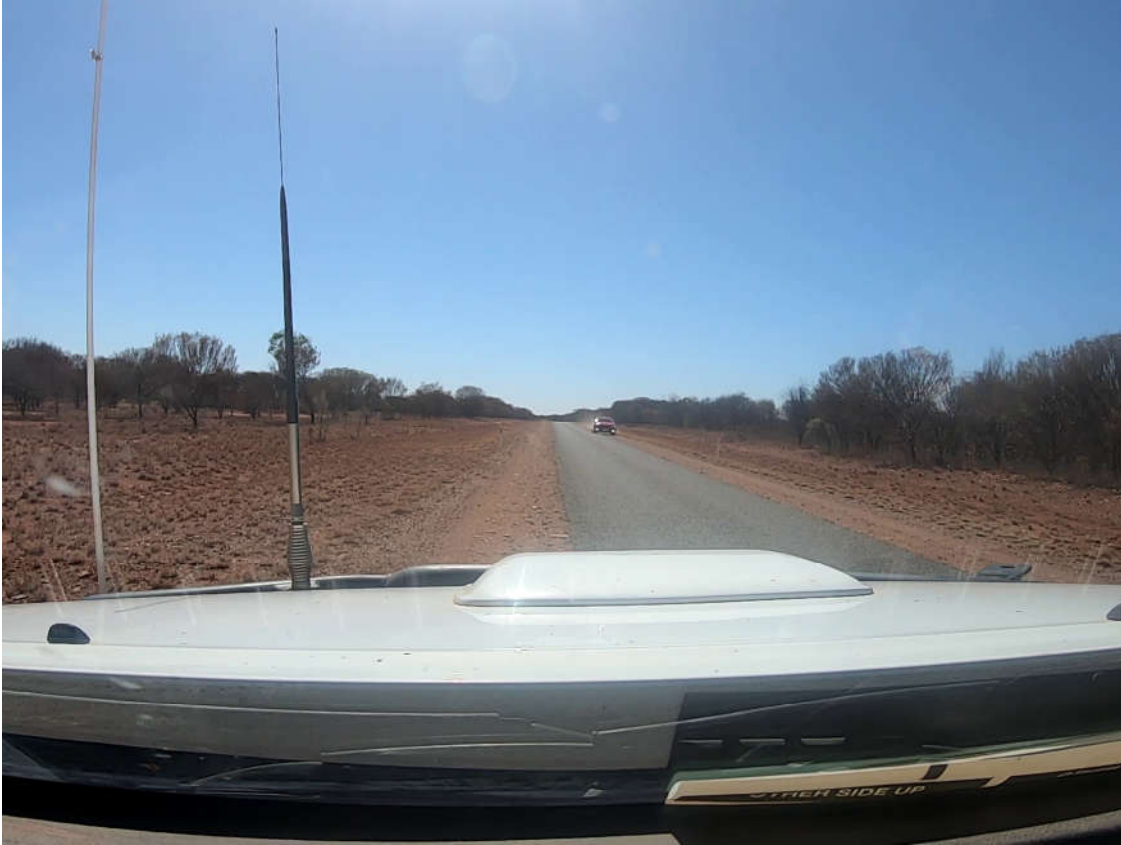
Photo 5 – Large drop off from seal to shoulder
