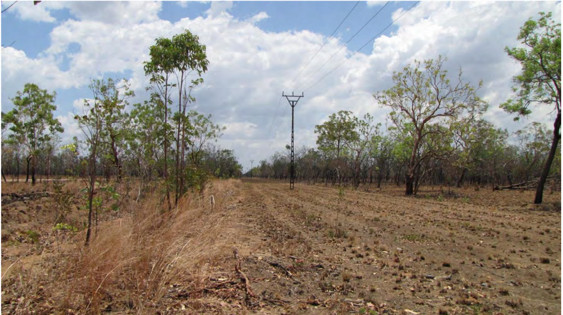
Figure 24: Powerline easement and Central Arnhem Highway (left) through Northern Crested Shrike-tit habitat
