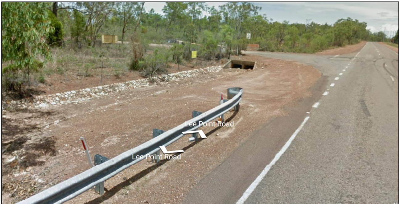
Figure 10. Entry road to 2CRU
