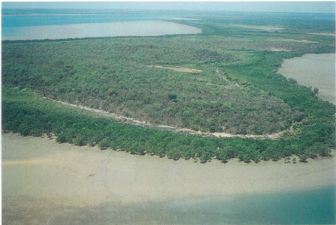
Aerial view of southwestern tip of Wickham Point peninsula - the main location of the proposed LNG plant. The main jetty will extend from the point (front right hand of photo) and the majority of the plant will be located behind the main rocky ridge (to left). The mangrove zone separating the western hinterland island from the eastern can be seen at centre right.
