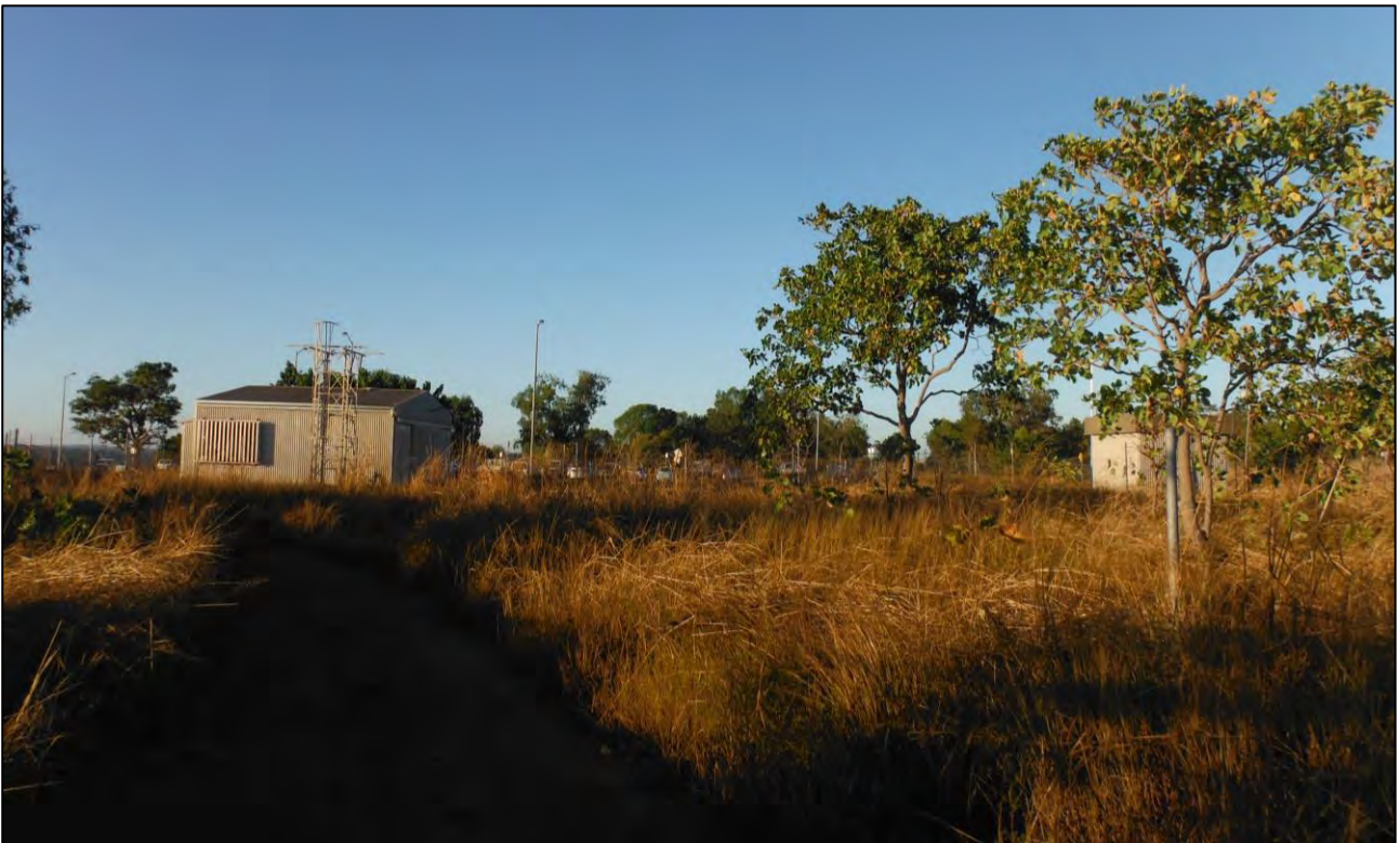
Figure 2-3 Existing abandoned building on Lot 50 and adjacent land – predominantly cleared
