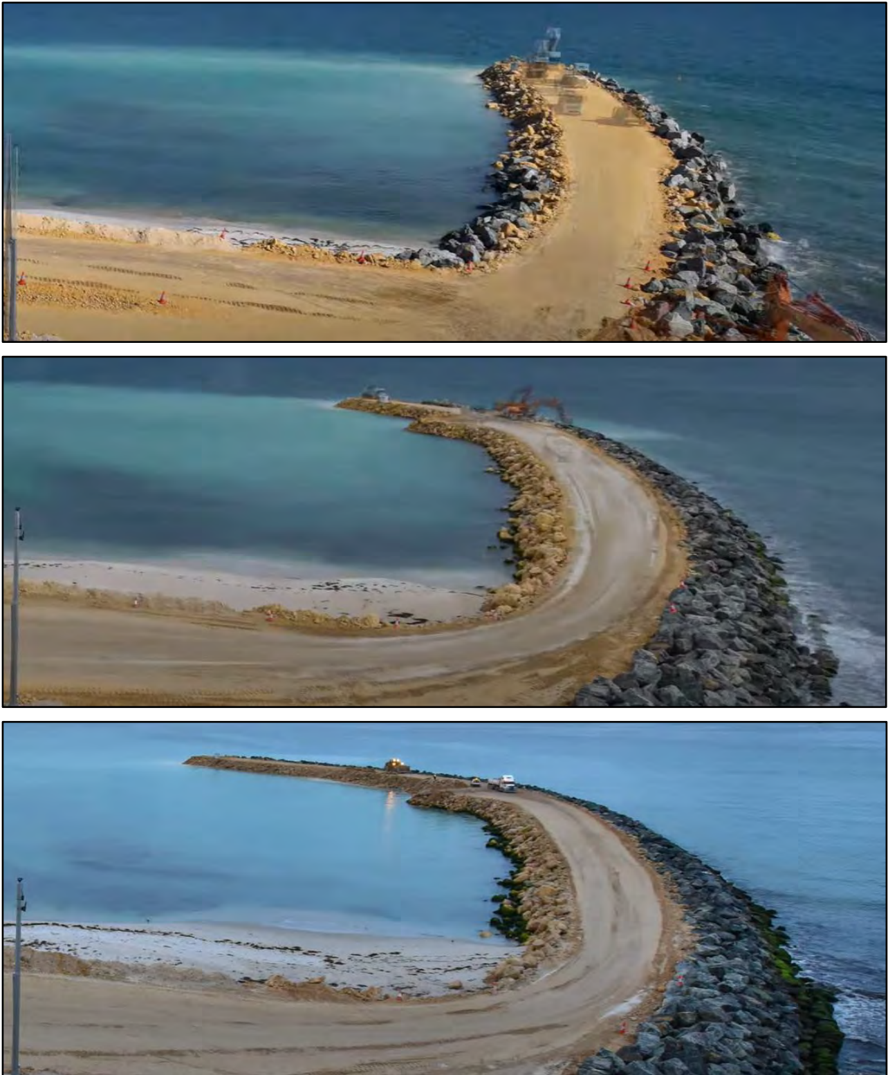
Figure 3-3 Example of staged breakwater construction (Ocean Reef Marina – DevelopmentWA, 2021)
