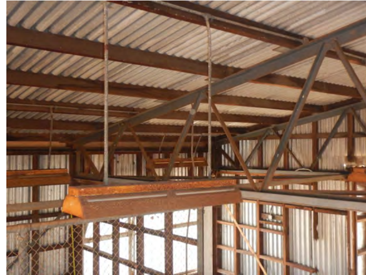
Photo 6 HW purlins, bolted truss top chord
