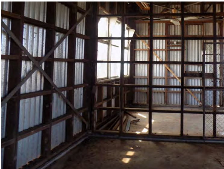
Photo 9 HW external studs wall framing
