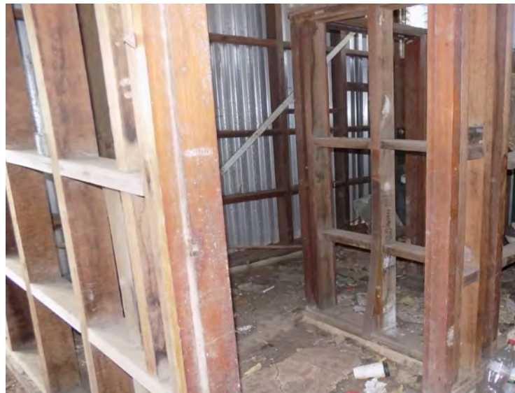
Photo 10 Typical HW internal wall framing
