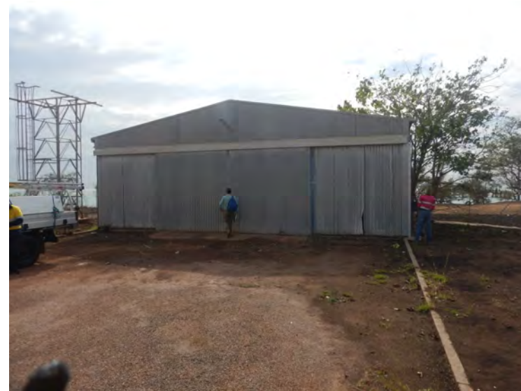
Photo 4 Entrance to/western wall of Radio Australia shed building
