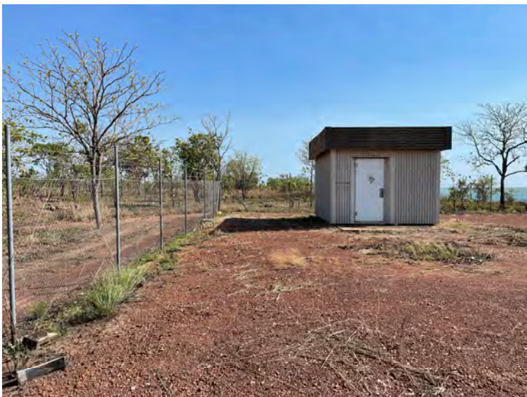
Photo 11 Existing SMALL BUILDING found north west corner of the site
