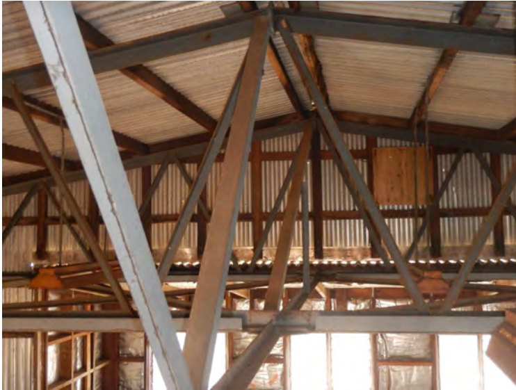
Photo 5 Steel framed latticed framed truss
