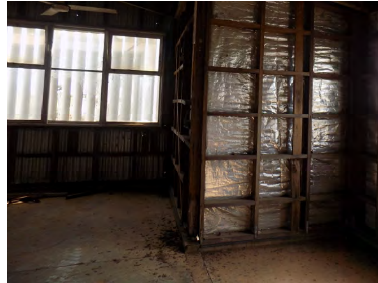
Photo 8 HW studs wall framing, sisalation
