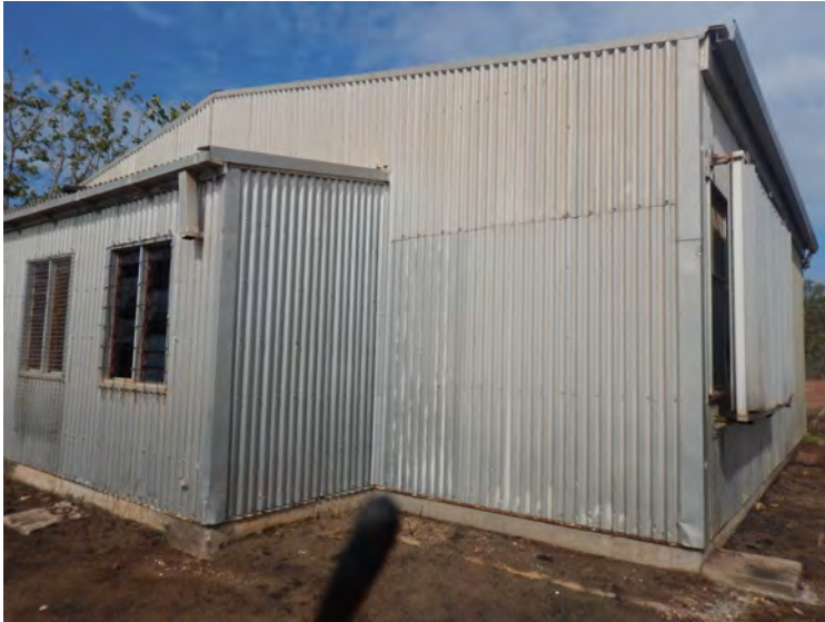
Photo 3 Eastern wall of Radio Australia shed building
