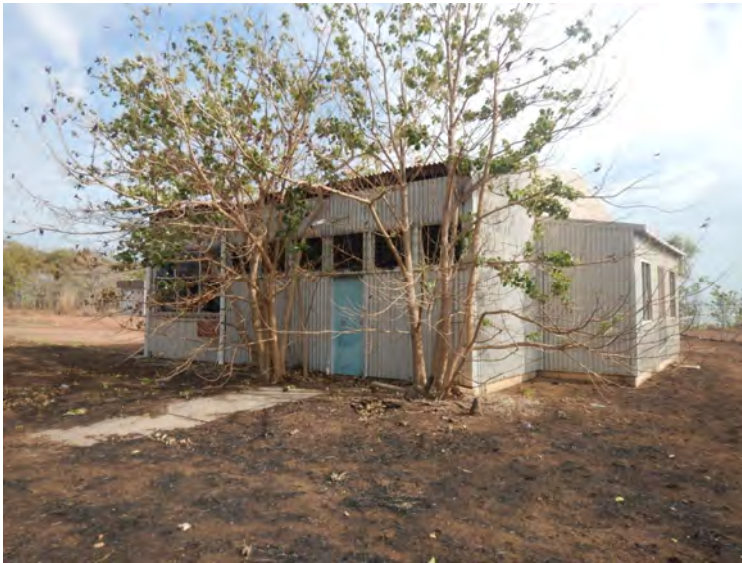
Photo 1 Southern Wall of Radio Australia shed building
