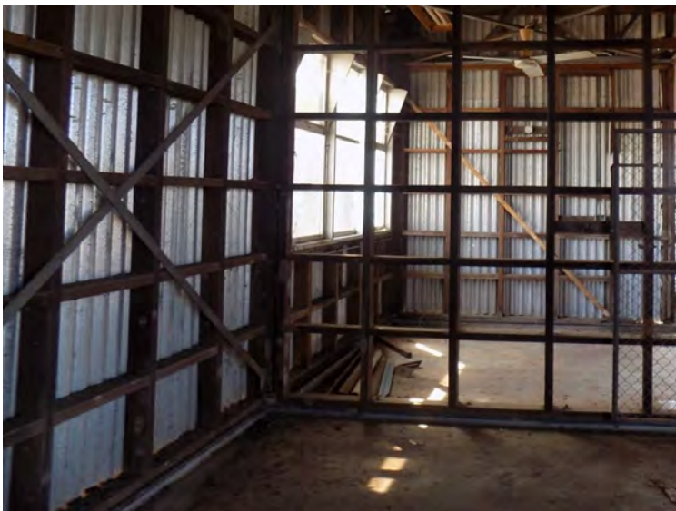
Photo 9 HW external studs wall framing
