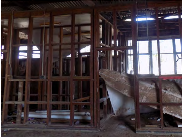
Photo 7 HW internal studs wall framing
