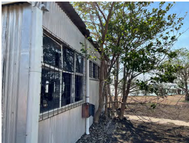
Photo 13 Southern external wall
