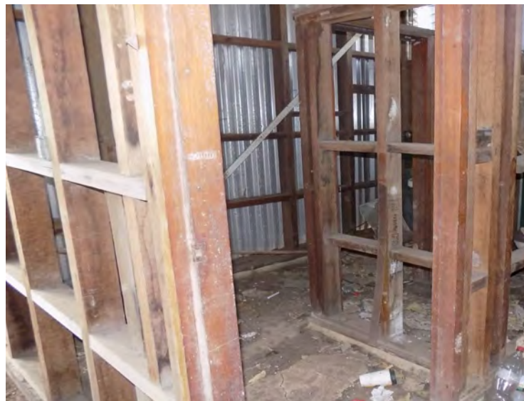
Photo 10 Typical HW internal wall framing
