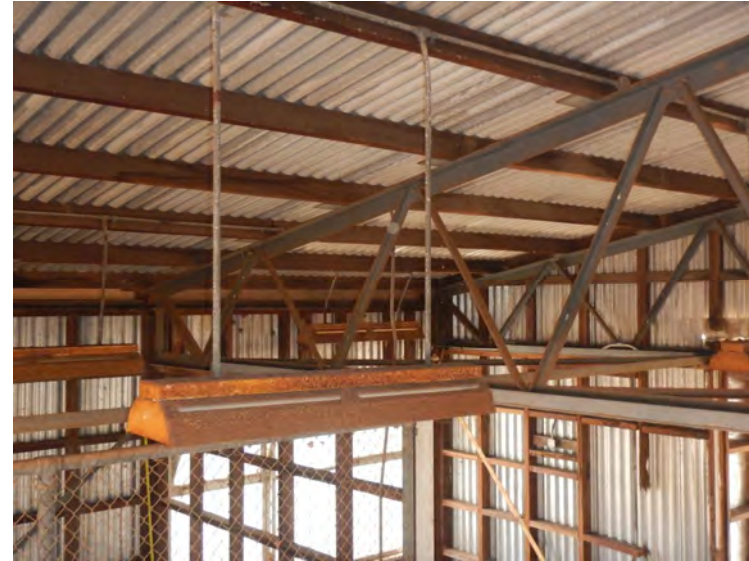
Photo 6 HW purlins, bolted truss top chord
