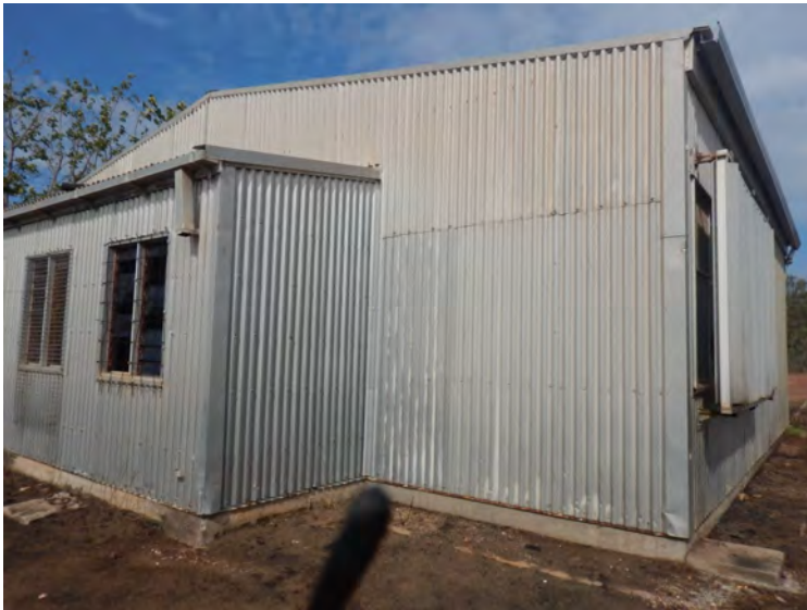
Photo 3 Eastern wall of Radio Australia shed building
