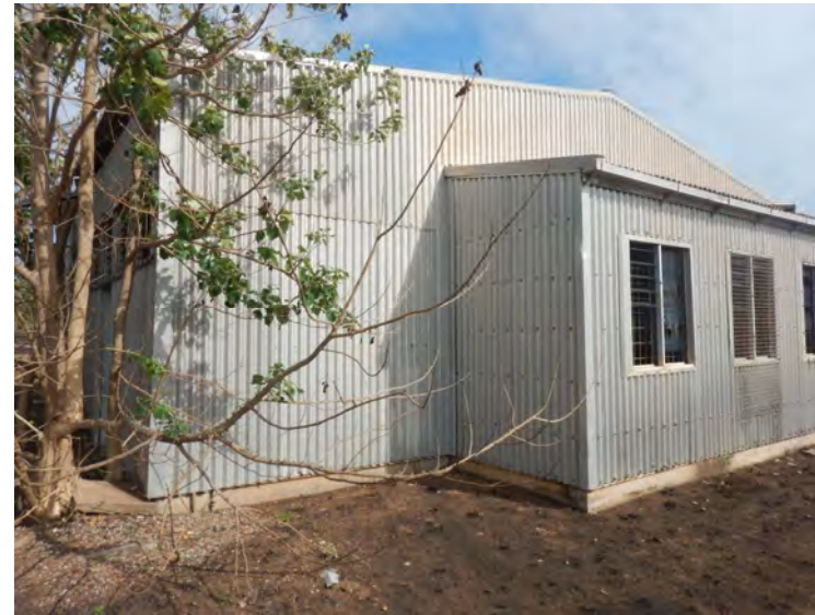
Photo 2 Eastern wall of Radio Australia shed building
