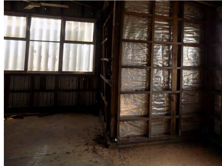
Photo 8 HW studs wall framing, sisalation
