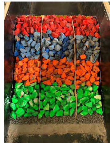
(l) 6-10T primary armour completed
