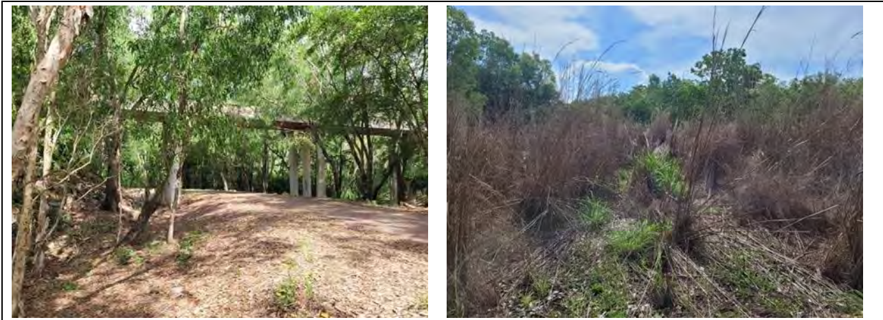
Figure 2-4. Images of the easement condition between the Manton Dam Wall and Stuart Highway
