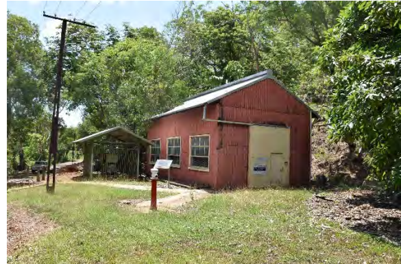
Remaining Steam Pumphouse 1
