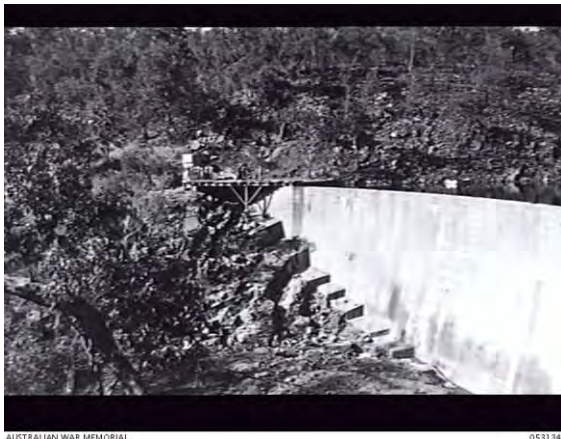
AUSTRALIAN WAR MEMORIAL 053134 Manton Dam 1939-1945
