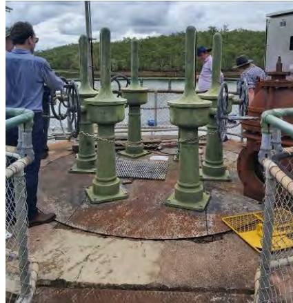
Remaining infrastructure on intake tower
