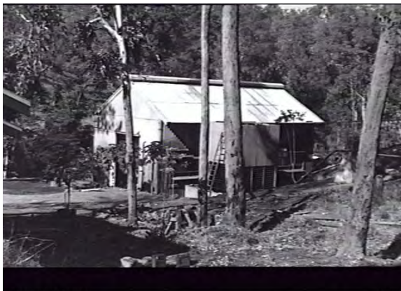
AUSTRALIAN WAR MEMORIAL Steam Pumphouse 2 - 1943
