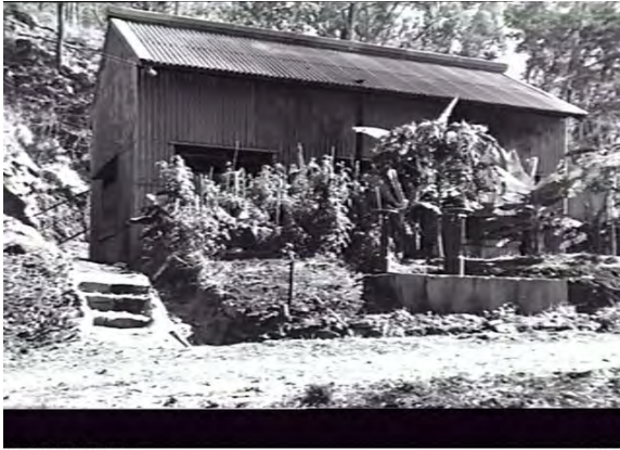
AUSTRALIAN WAR MEMORIAL Steam Pumphouse 1 - 1943
