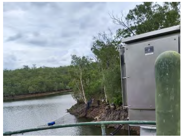
Remnants of boom system pylon footings
