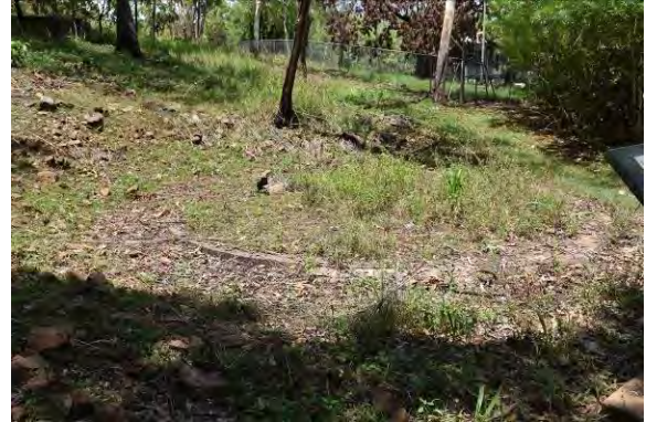
Remaining tank base
