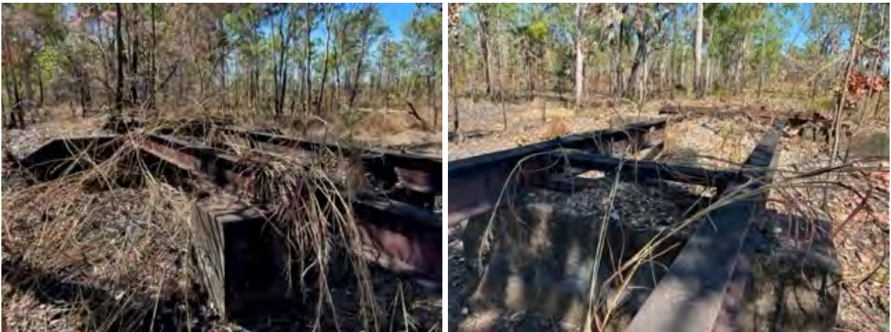
Figure 5-8. Photos of NAR Railway Bridge (ID 8 in Figure 5-9)
