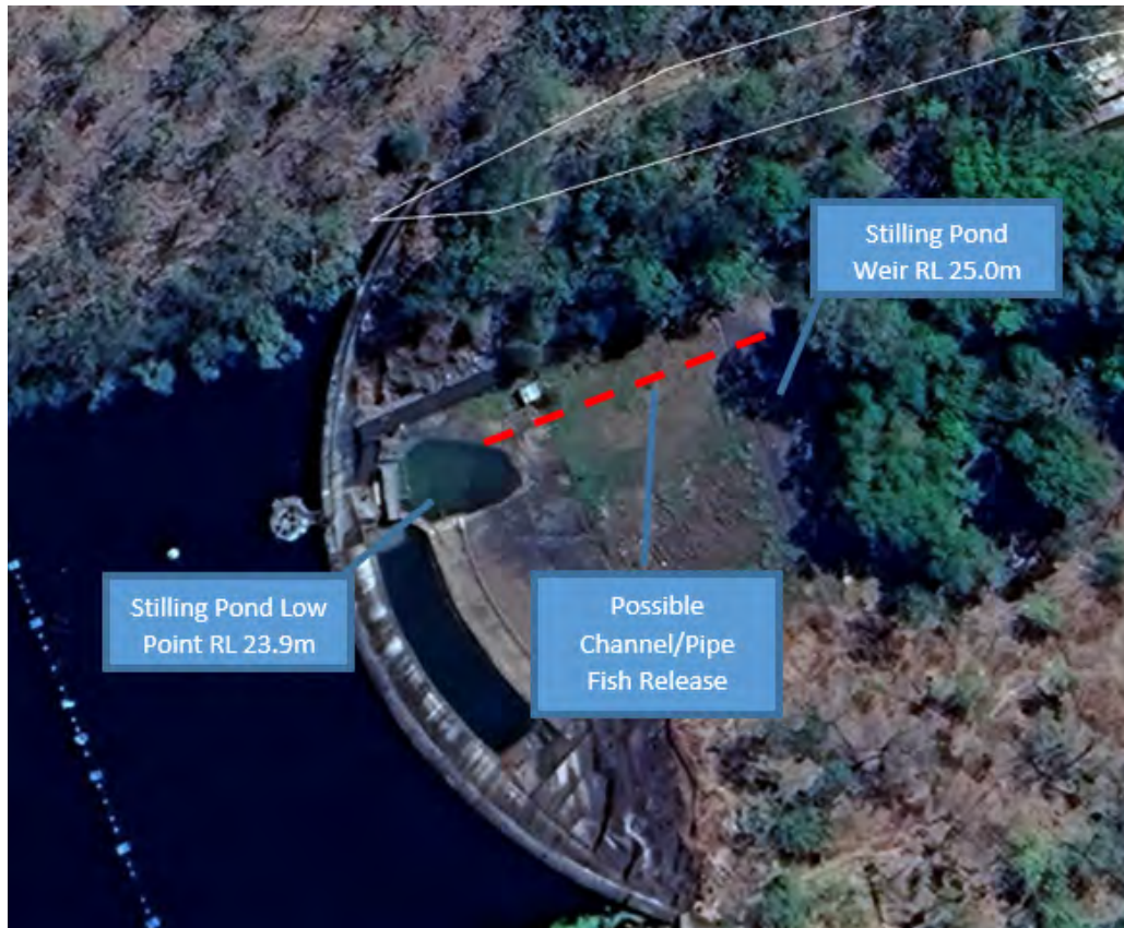
Figure 2-7. Location of stilling pond at Manton Dam wall and potential channel/pipeline route
