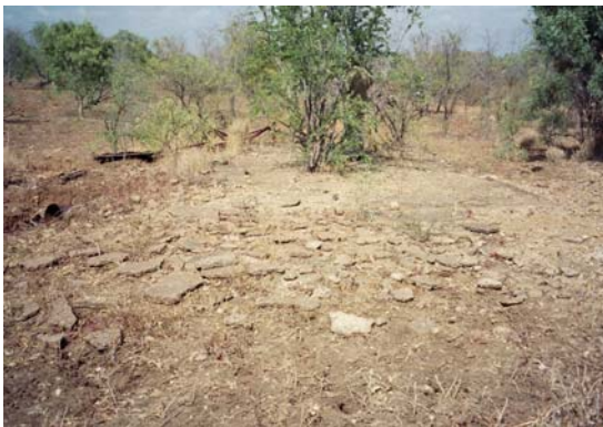
Photo 12. MRMH2, largest concrete floor
