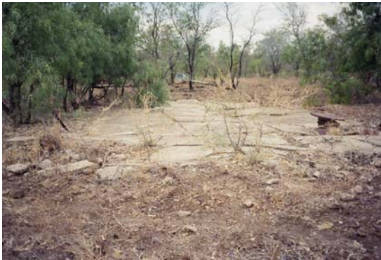
Photo 10. MRMH1, largest concrete floor
