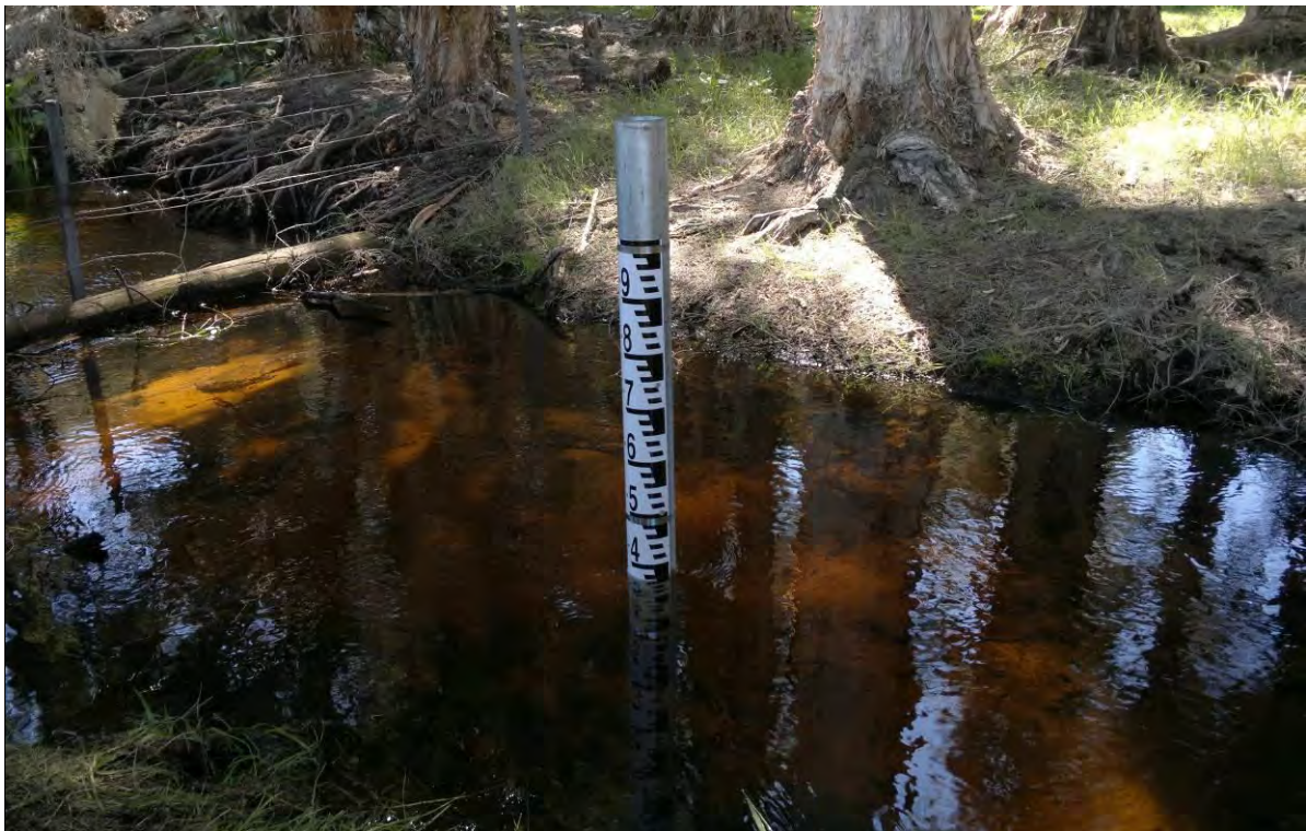
Figure 4-2: Example of surface water installation incorporating a stream gauge plate and internally-mounted water level instrument
