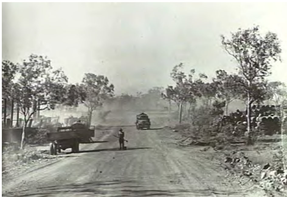
Figure 4.14 A convoy approaching a staging camp on the 'North-South Military Highway', 1943. Allied Works Council tar and bitumen boilers, left, were used in the resurfacing works (Source: Australian War Memorial, ID. 014400).
