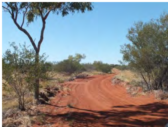
Figure 6.86 View east towards cleared and partially graded access road between borehole sample locations, mine pit area.
