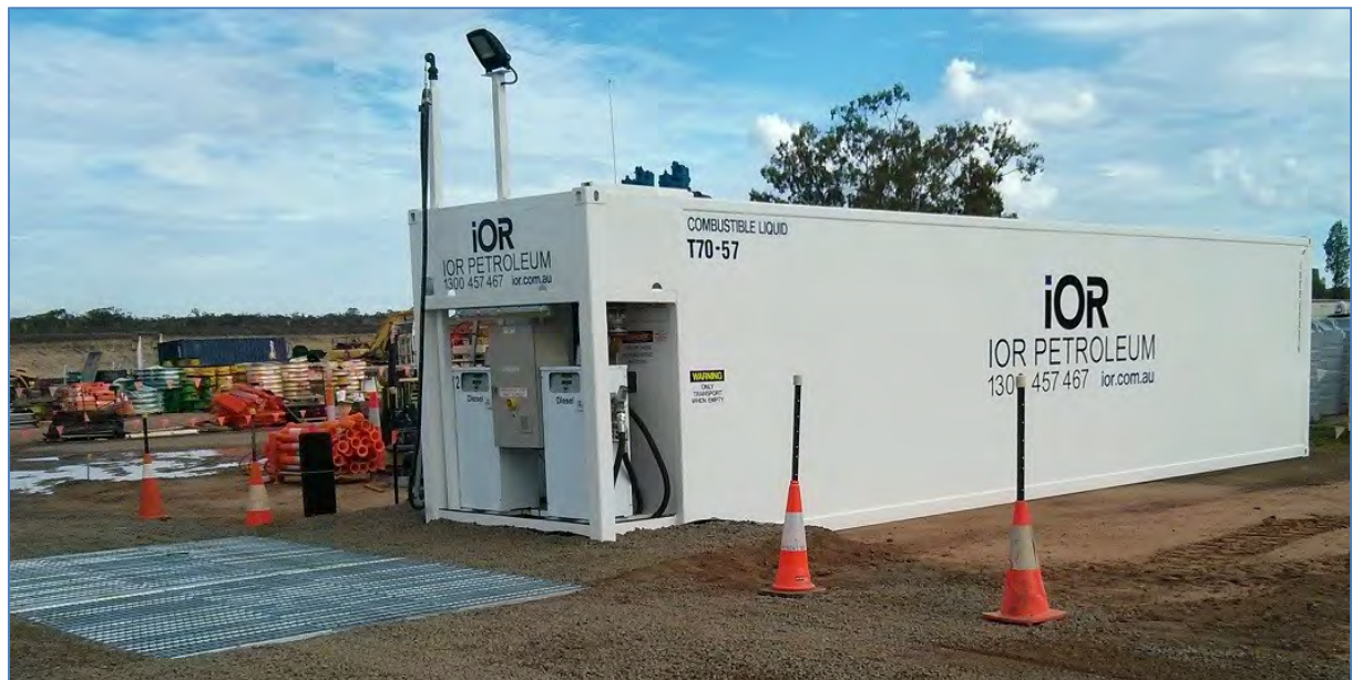
Plate 2-2 Example of 85,000 L self-bunded tank
