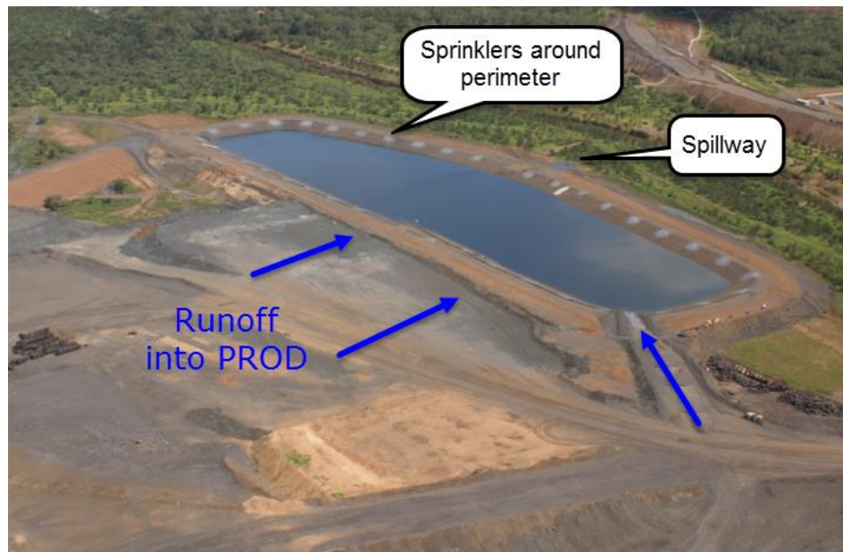
Figure 8-19 Aerial View of SEPROD
