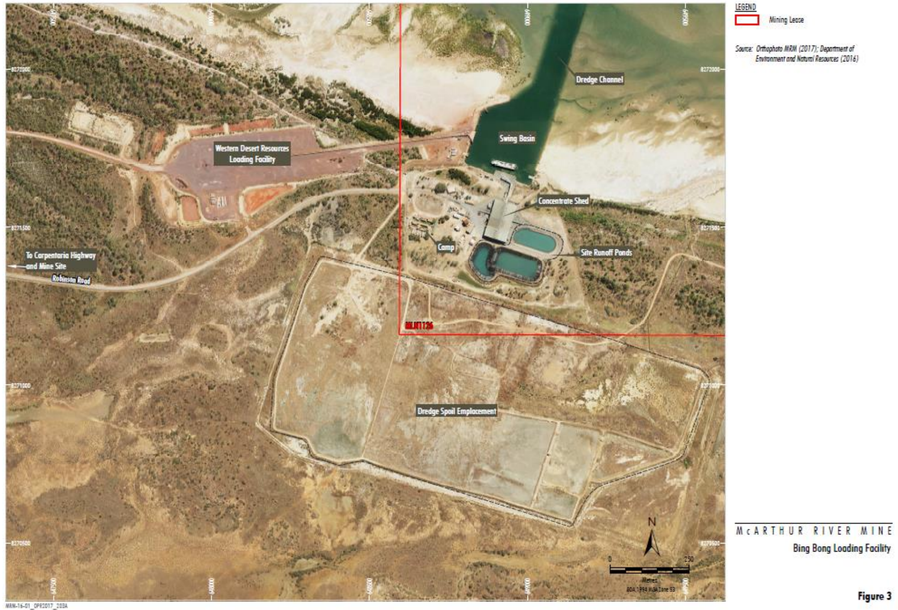
Figure 3 – Bing Bong Loading Facility
