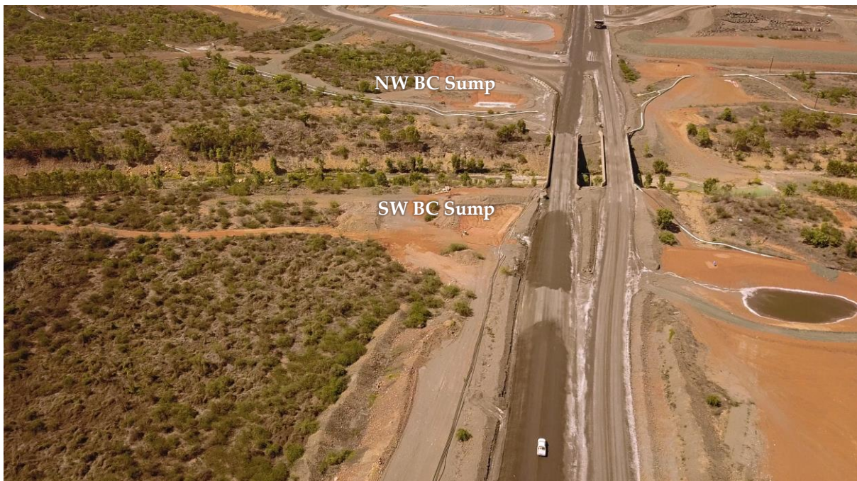
Figure 3-6 New Barney Creek Sumps
