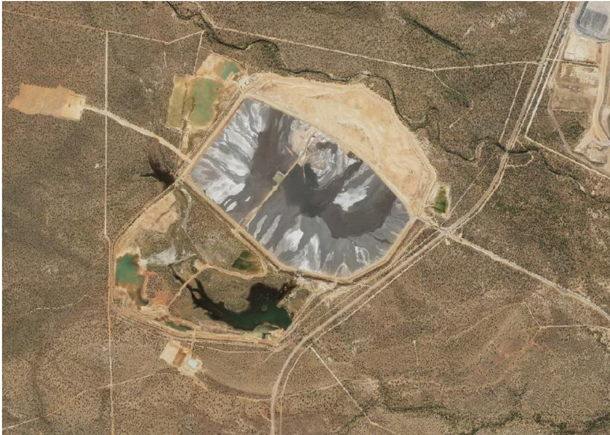
Figure 3-7 TSF as of June 2017 Showing Dry Large Tailings Beaches and Small Central Decant Pond
