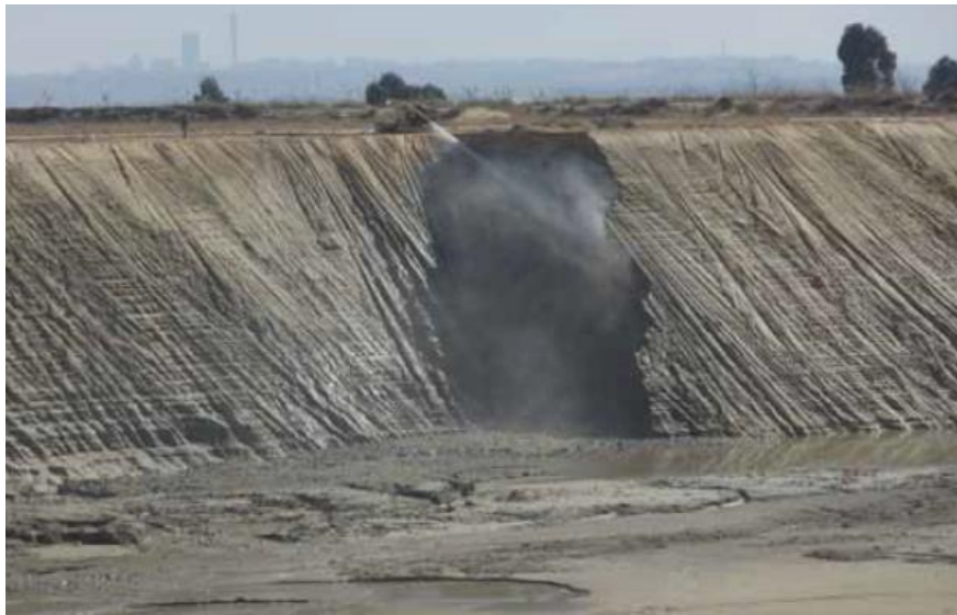
Figure 6-16 Example of Hydraulic Monitor Operation
