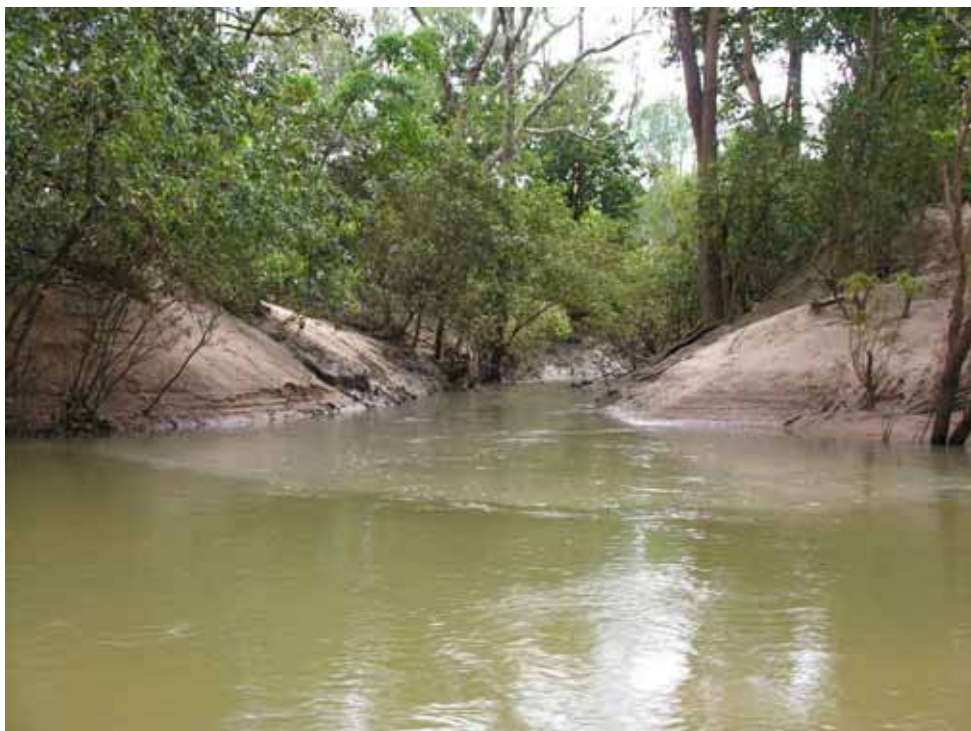
Plate 4.10 Unstable Steep Sand Banks at the Mouth of Barney Creek
