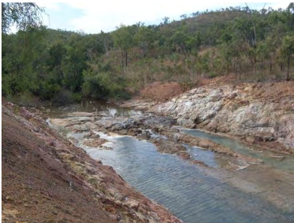
Photo 21 Horseshoe Creek existing upstream diversion
