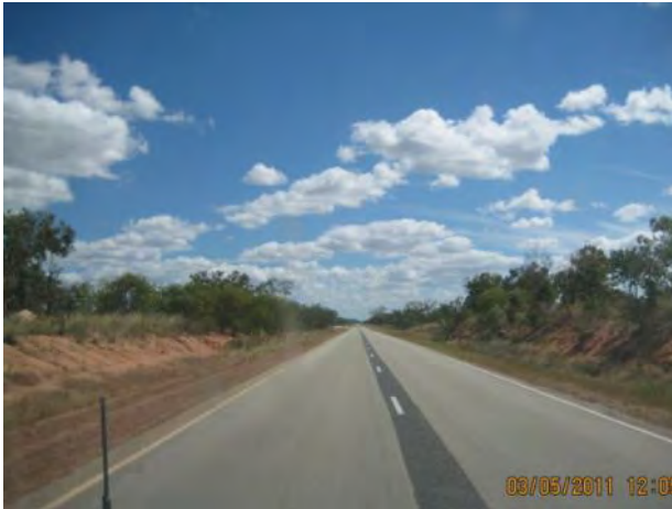
Figure 3 Stuart Highway typical two-lane two-way cross section
