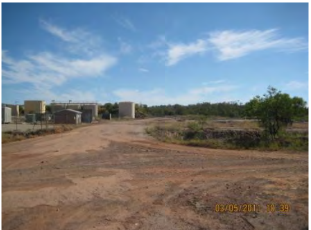
Figure 10 Internal Mine Roads, unsealed sections of roads
