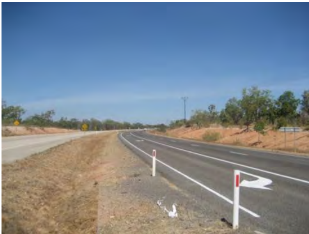
Figure 11 Sight distances at the Stuart Highway / Edith Falls Road intersection, view to south on Stuart Highway
