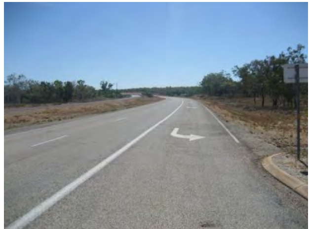
Figure 12 Sight distances at the Stuart Highway / Edith Falls Road intersection, view to north on Stuart Highway
