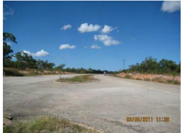
Figure 4 Stuart Highway dual carriageway cross section at Edith Falls Road intersection, view to south
