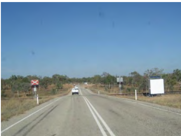
Figure 15 Edith Falls Road level crossing, view to west
