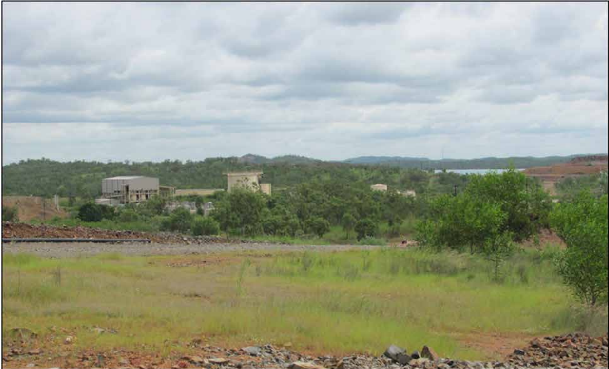
Plate 2-7 Existing Mine Site Processing Plant and Lime Kiln
