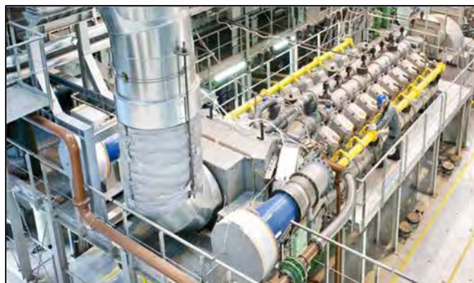
Figure 2-11 MAN 20V35 / 44 SG Recip. Engine
