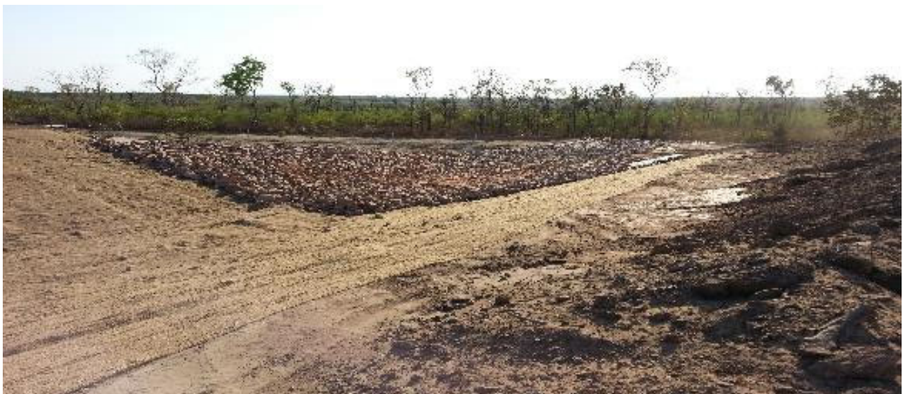
Plate 3-5 Example of Diversion Channel and Rock Armoured Outlet.
