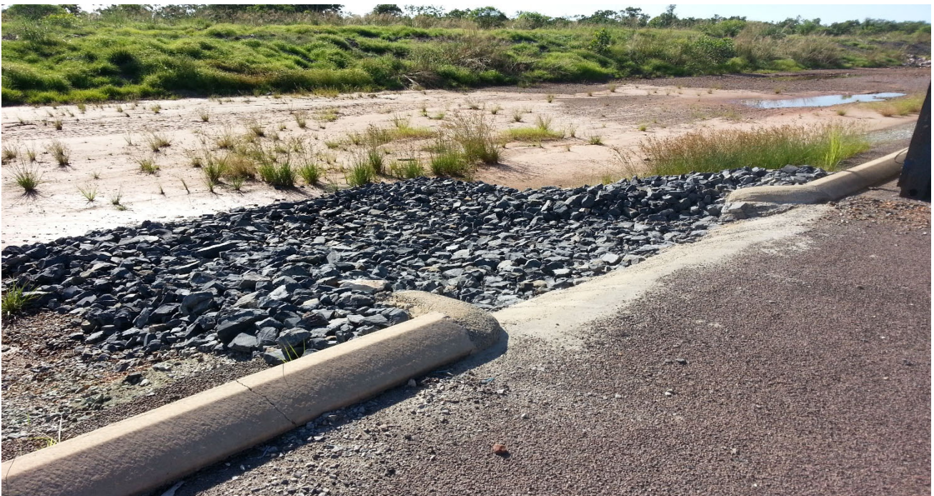
Figure 3-8 and Plate 3-8 Example of Small Rock Shute and Dissipater off a Hardstand.
