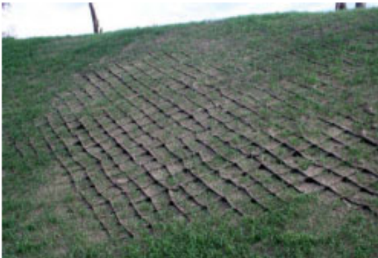
Plate 3-1 An example of cellular confinement system used to restrict gravel movement on a carpark.
