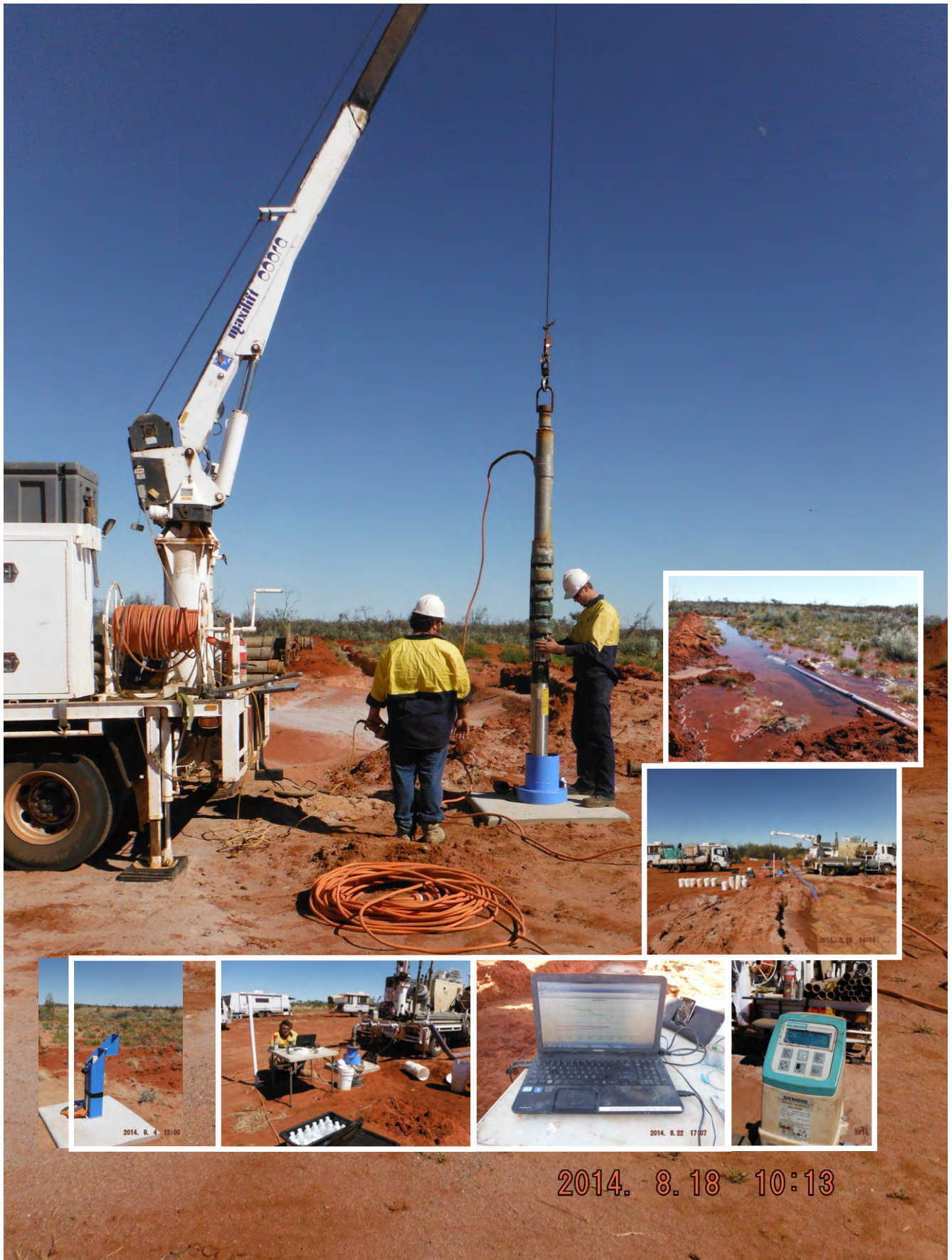
Constant Rate & 4 stage pump test Bore RC # 31 (bore site P1)
