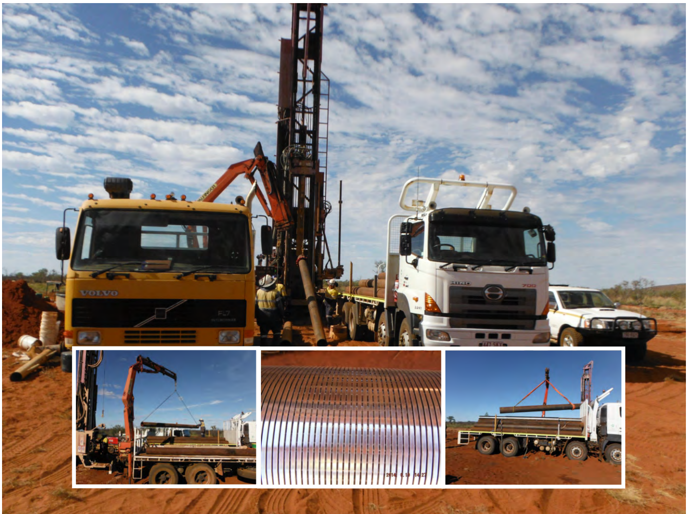
L2 Drillers casing Arafura Reaphook Paleochannel production bore P1
