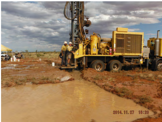
Diverse Resources Group drilling PB2 a 250 mm ID steel cased gravel packed bore with inline stainless steel screens using Pac R mud circulation using a T3W Drilling Rig
