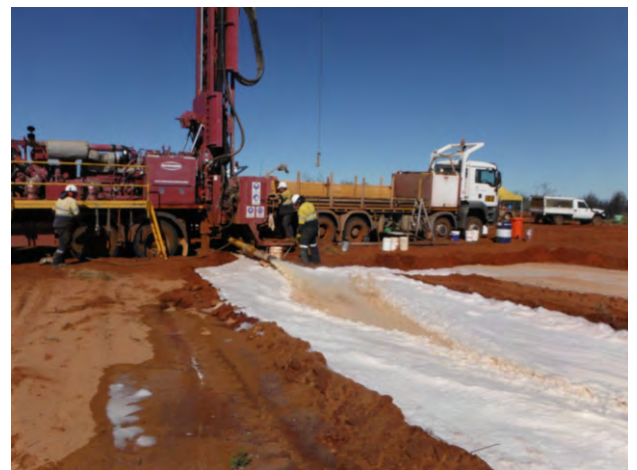
L2 Drillers completed the majority of the stage 2 water bores using a Schramm Drilling Rig
