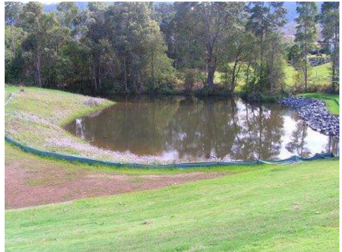
Figure 2-21. Photograph of detention basin
