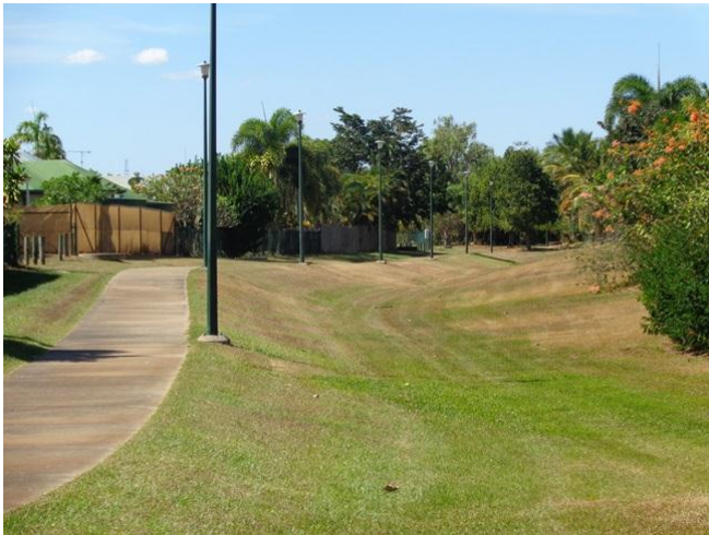
Figure 2-20. Photograph of grassed swales
