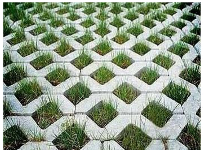
Figure 2-24. Photograph of porous pavement
