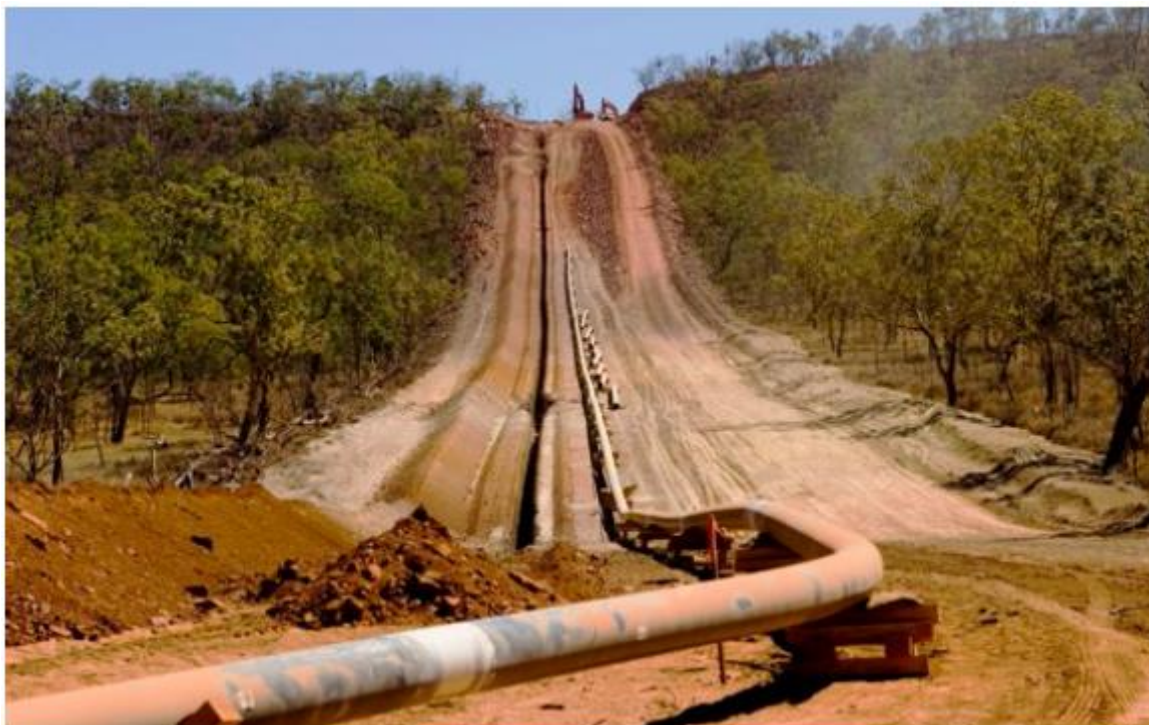
STRINGING THE BONAPARTE PIPELINE 2006
