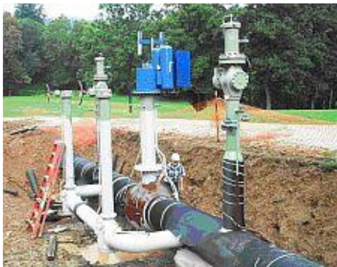
Figure 7: Typical MLV Assembly
